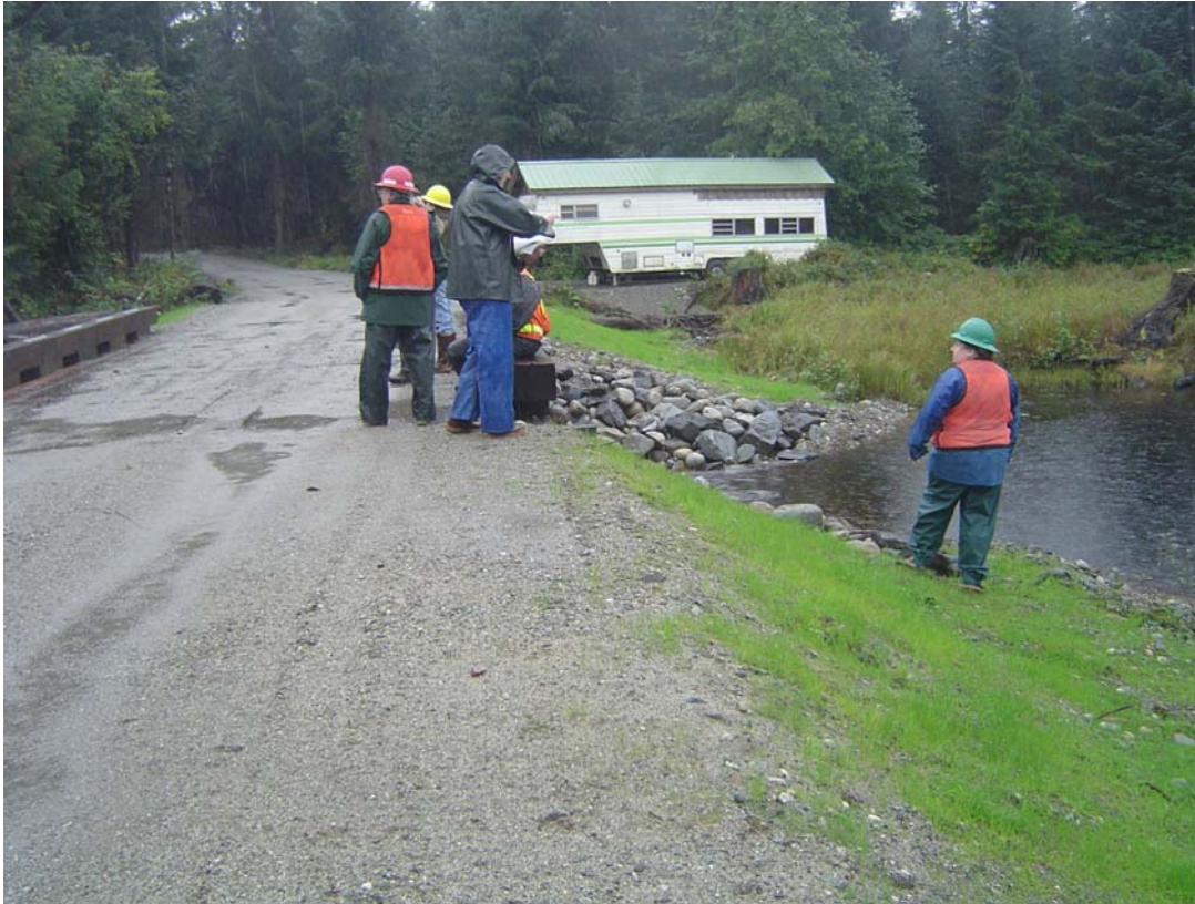
Photo 1. Site E, Bridge at Road 6256 MP 3.543. Photo taken looking towards Thomas Bay. Note well-established vegetation (BMP 14.8). Note placement of riprap along banks (BMP 14.17), and rock weir partially visible was used to maintain the preconstruction pond elevation (BMP 12.5).
