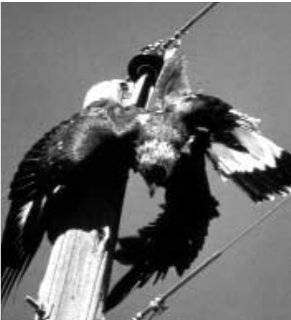
Agents worked with electric power companies in Arizona and New Mexico to prevent the electrocution of raptors and other protected birds. Peter Carboni/USFWS
