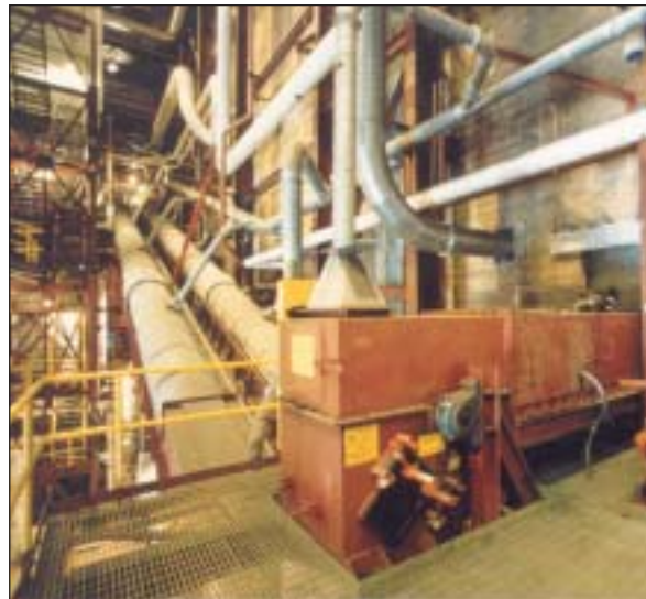
Coal and sorbent conveyors can be seen just after entering the Tidd plant.
