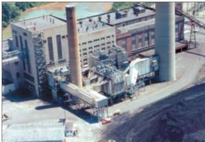
Bechtel's demonstration showed that 50% \text{SO}_2 removal efficiency was possible using CZD/FGD technology. The extended duct into which lime slurry was injected is in the foreground.
