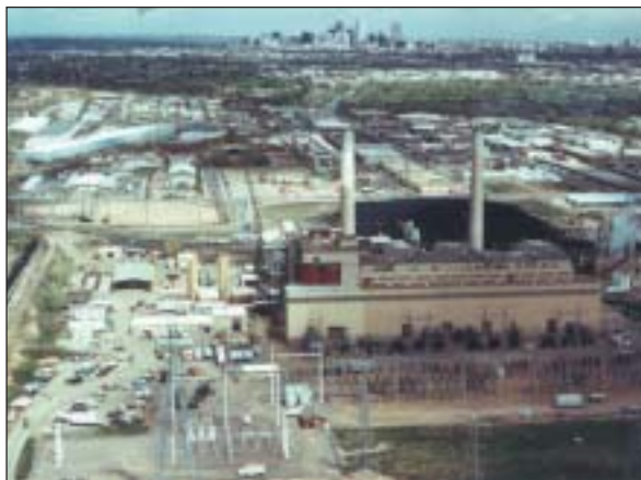
Public Service Company of Colorado demonstrated low-NO x burners, in-duct sorbent injection, and SNCR at Arapahoe Station near Denver, Colorado.
