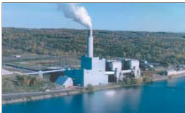
Milliken Station served as the host for two CCT Program projects demonstrating advanced environmental controls.
