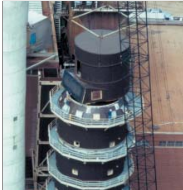
LIFAC reactor being installed in Richmond, Indiana.
