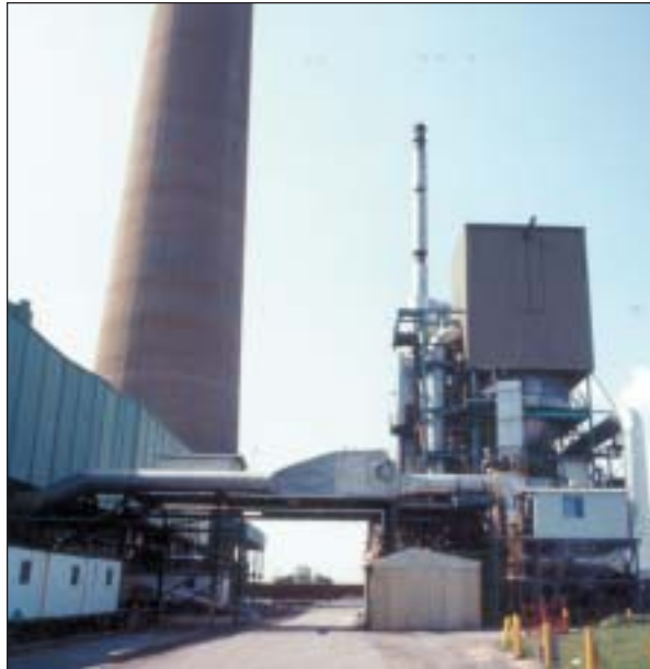
The 10-MWe AirPol gas suspension absorption demonstration unit.
