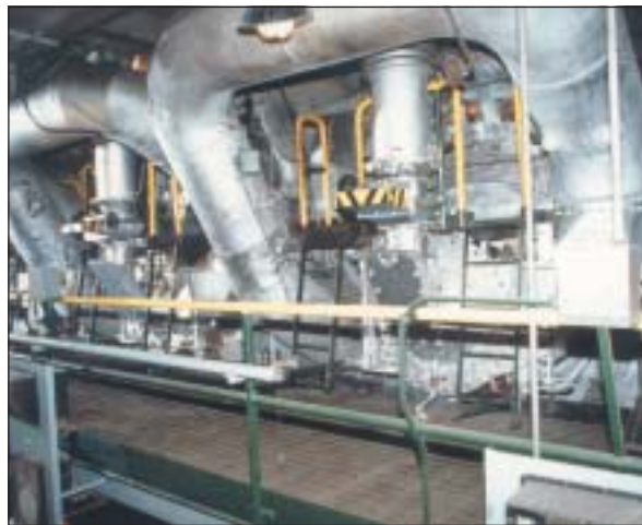
Air and coal feed for coal reburning in a cyclone boiler at the Nelson Dewey Station.
