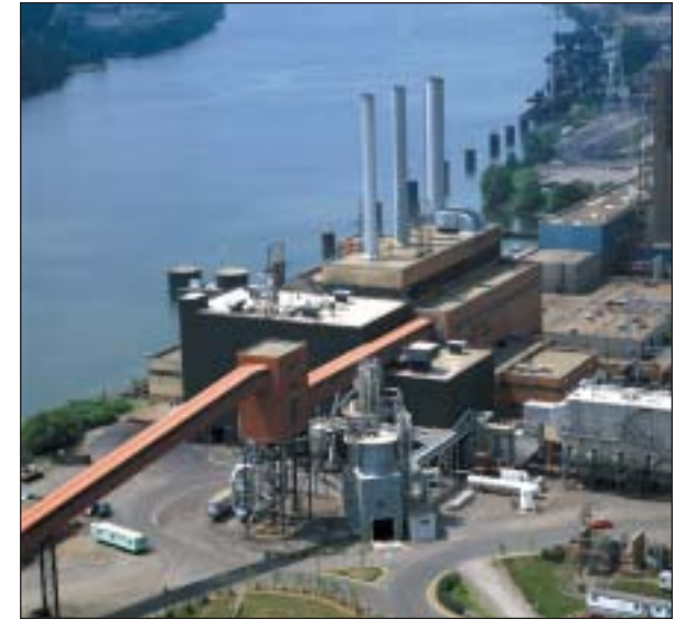
Tidd PFBC Demonstration Project (The Ohio Power Company)—1991 Powerplant Award presented by Power magazine.
