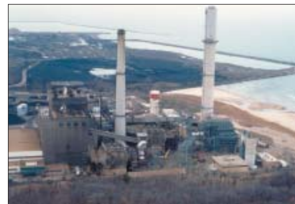
Advanced Flue Gas Desulfurization Demonstration Project (Pure Air on the Lake, L.P.)—1993 Powerplant Award presented by Power magazine.
