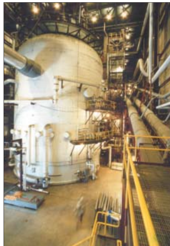
Pressurized fluidized-bed combustion, like that demonstrated at Ohio Power Company's Tidd Plant, is starting to see global commercialization.
