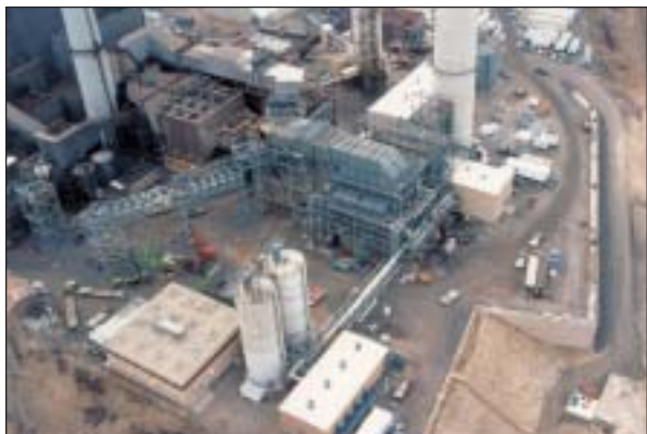
The Pure Air on the Lake, LP AFGD absorber module at base of stack with sorbent silos in the foreground.
