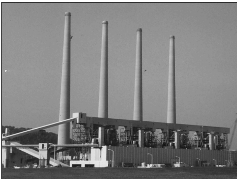
▲ Dayton Power and Light Company's J.M. Stuart Plant hosted the successful demonstration of LNCB® technology.
