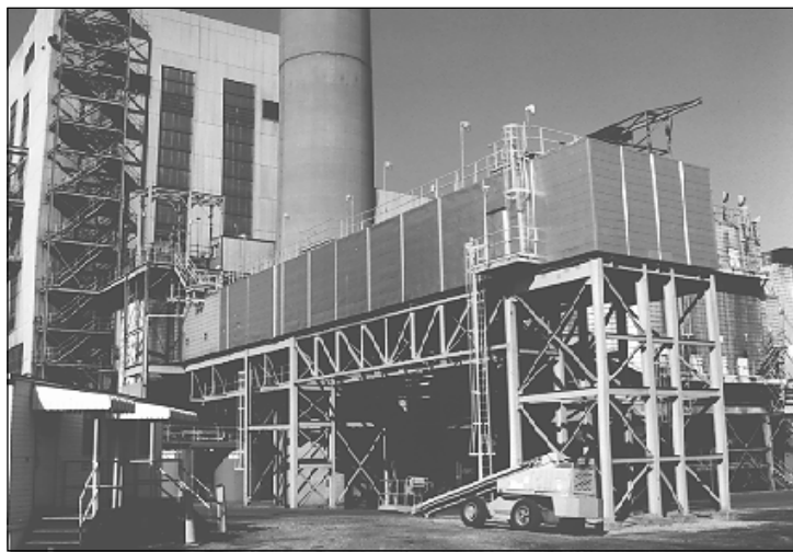
▲ Bechtel's demonstration showed that 50% SO 2 removal efficiency was possible using CZD/FGD technology. The extended duct into which lime slurry was injected is in the foreground.
