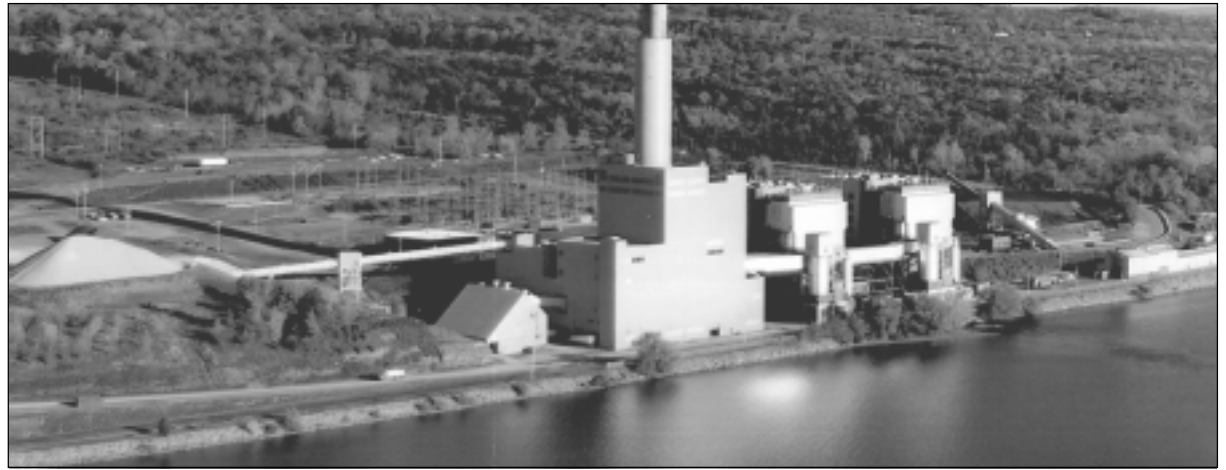
▲ New York State Electric & Gas Corporation's Milliken Station is hosting the demonstration of a combination of unique SO 2 and NO x control technologies.
