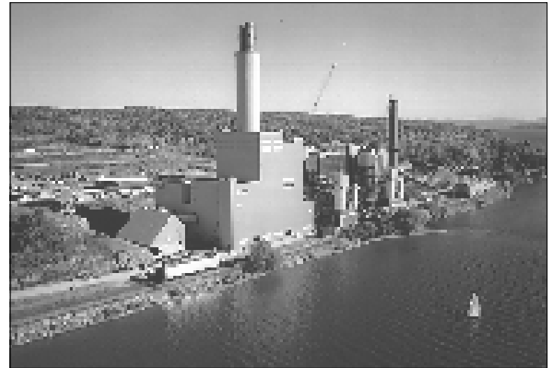
▲ New York State Electric & Gas Corporation's Milliken Station used the S-H-U scrubber to achieve Phase I SO 2 compliance.
