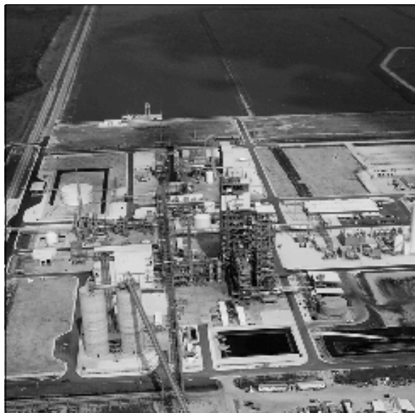
▲ Tampa Electric Company's Polk Power Station Unit 1, a 250-MWe IGCC greenfield installation, is currently in operation. It is one of the world's cleanest and most advanced coal power plants.
