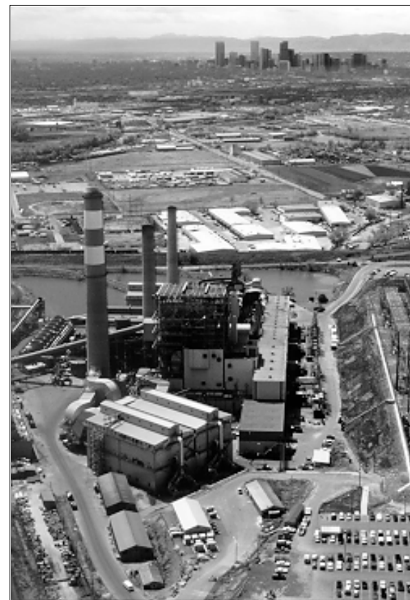
▲ The Public Service Company of Colorado has retained the gas-reburning and low-NO x burner system for commercial use.
