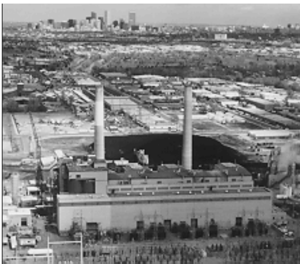
▲ Public Service Company of Colorado demonstrated low-NO x burners, induct injection, and SNCR at Arapahoe Station near Denver.
