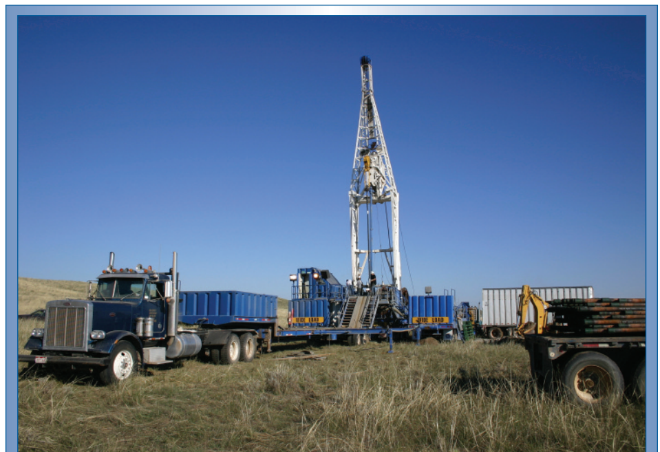
Figure 1. Rapid mobilization and demobilization of lightweight, easily transportable coiled tubing rigs is one of the keys to sharply reduced costs in microhole drilling.
