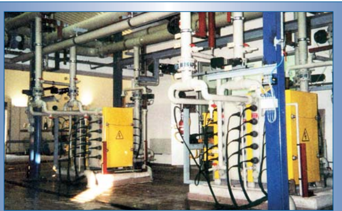
Figure 4. A commercial electrodiagnosis system for water treatment. (Photo courtesy of Ameridia, a division of Eurodia Industrie S.A.)
