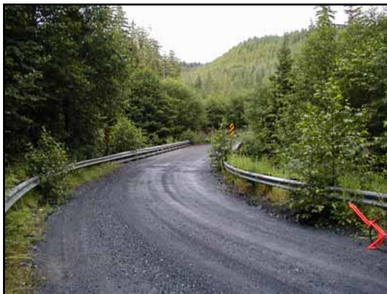
Typical ML 3 arterial road surfaced with aggregate.
