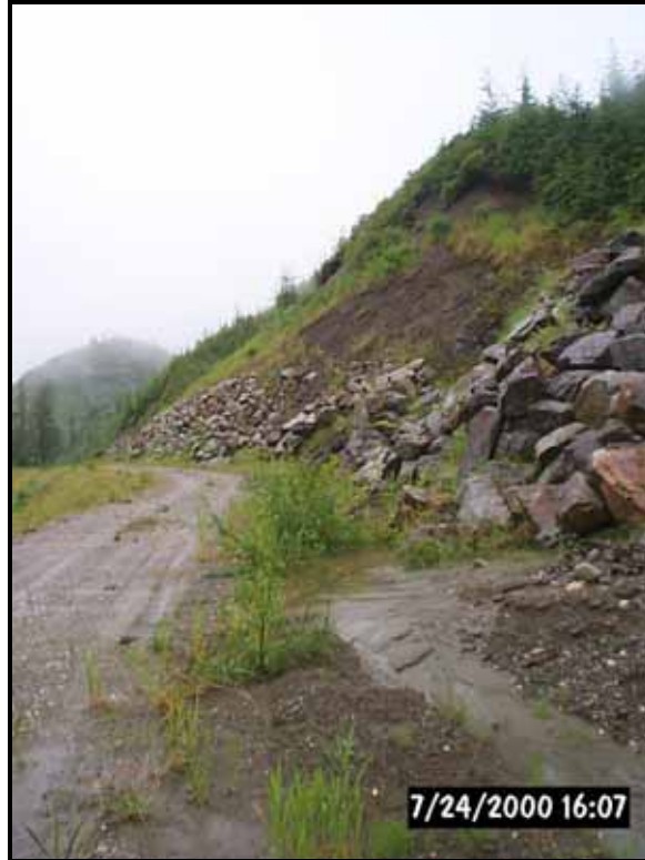
Riprap to control a cut-slope failure
