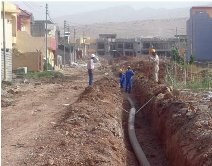
The Masike to Jami Bini water network will provide a reliable water supply for approximately 65,000 people, improving the quality and quantity of safe drinking water in the area. The $1.5 million project also provides collateral benefits of increasing water pressure, which reduces contamination; filling existing water storage tanks; and slowing aquifer depletion.
