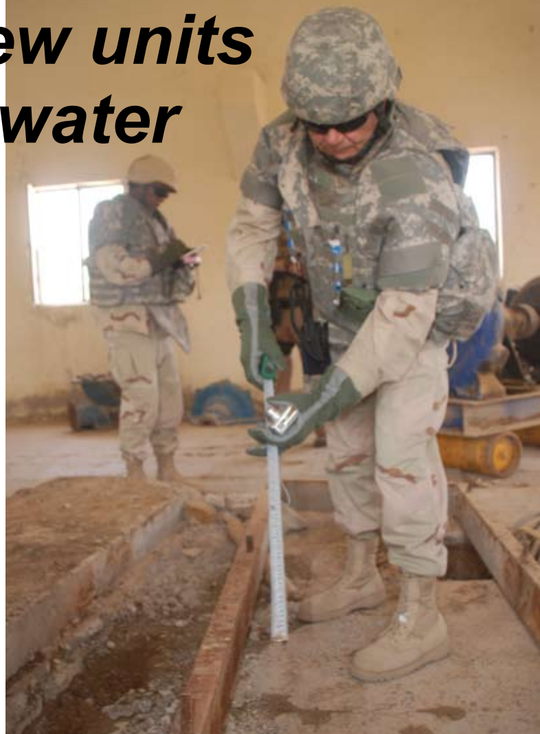
John Morgan takes a measurement, right, as Toni Graves notes the condition of a motor and pump.
