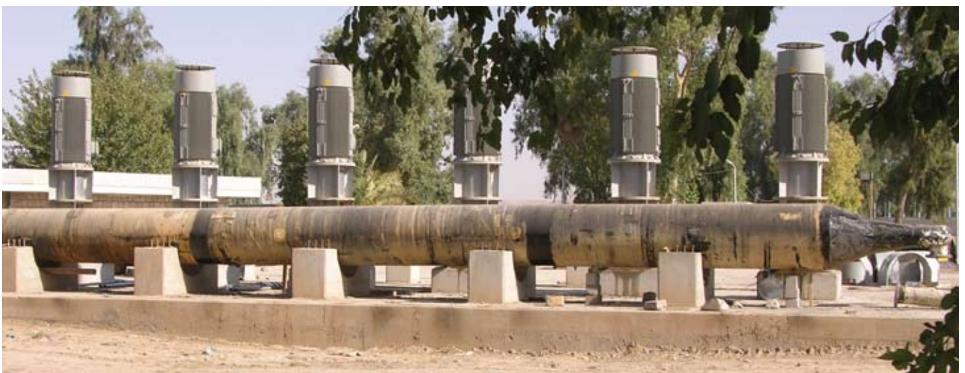
The Dibbis pump station increases the supply of potable water to 24 million gallons daily for the citizens of Kirkuk Province. The $8.2 million project included six new vertical pumps, above.
