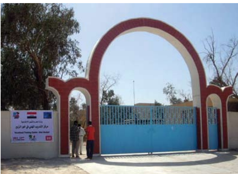
The new main entrance gate at Khor Al-Zubair tech center, which supports the needs of 600 students.
