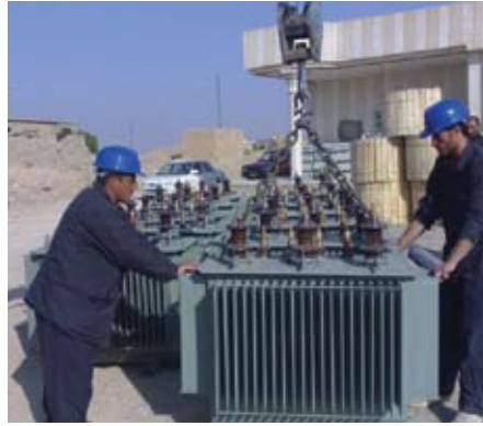
Contractors prepare to hoist a 250 kVA transformer for placement on new power poles in Tuz, Iraq.
