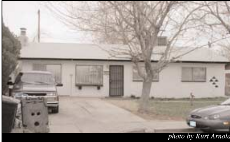
The front of Marie Fields' home before volunteers began any work.
