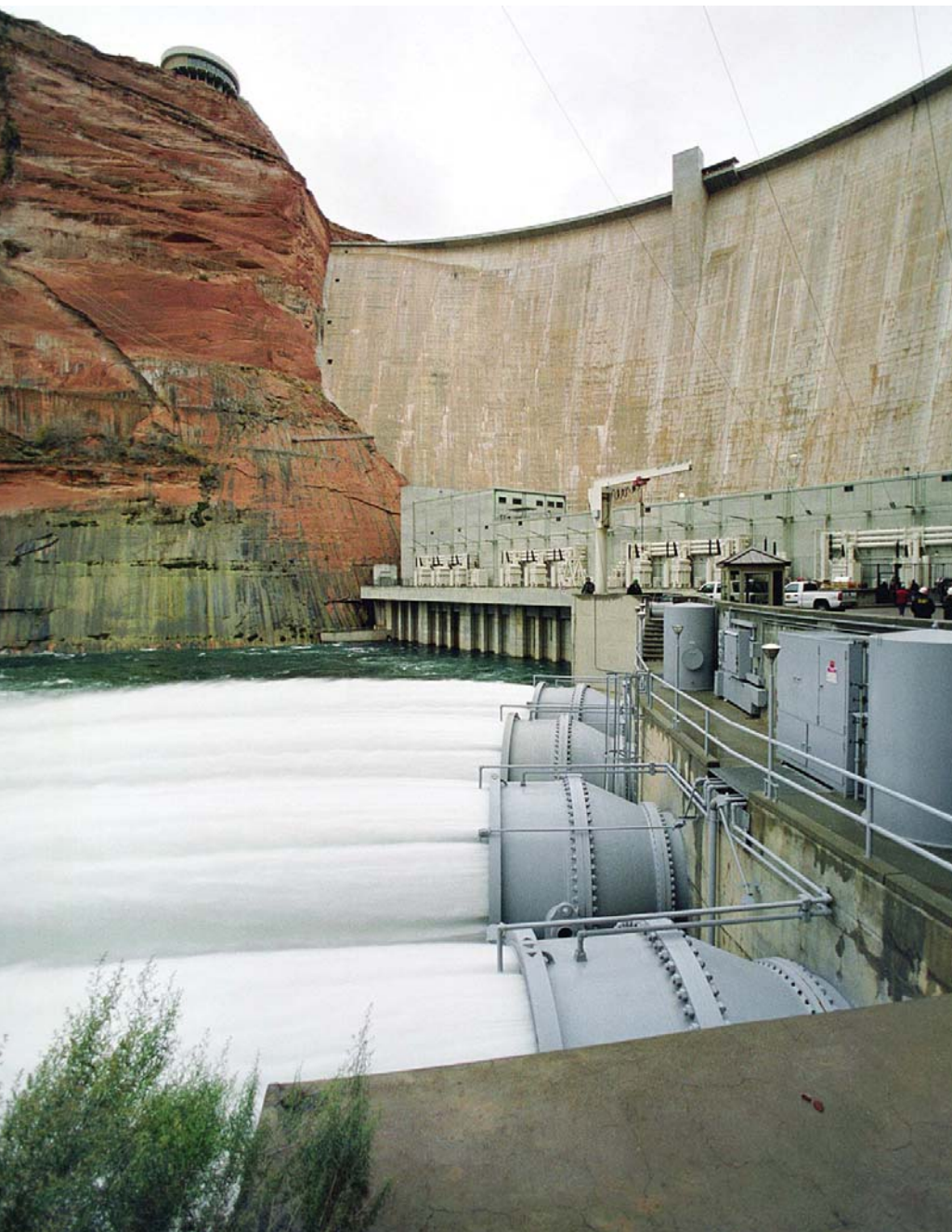
Figure 1. In 1996, dam operators sharply increased water releases from the Glen Canyon Dam on the lower Colorado River. The adaptive management experiment increased water flows to 45,000 ft 3 /s (1,260 m 3 /s) for one week in an effort to rebuild sandbars using sand from existing channel eddy deposits. This successful experiment was repeated in 2004, pictured here.
