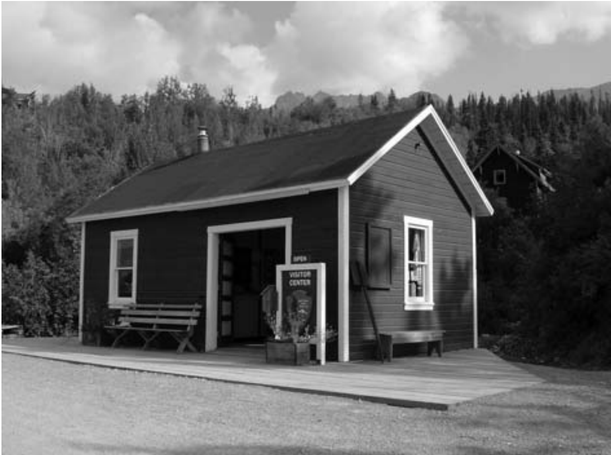
Figure 3. The former train depot in Kennecott currently serves as a temporary visitor center. COPYRIGHT STEVE TAYLOR
