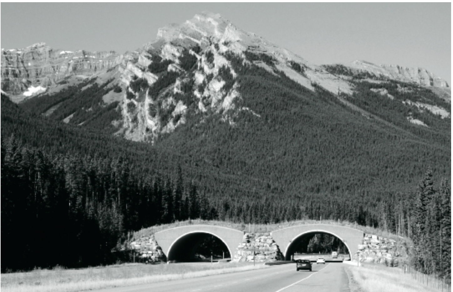
Figure 3. Banff National Park now has two multispecies overpasses that are part of a network of linkages designed to minimize the impacts of the Trans-Canada Highway on wildlife. Research has shown that human use of wildlife crossing structures has a greater impact on carnivore use than either placement or structural characteristics of the crossing. BRUCE LEESON, PARKS CANADA
