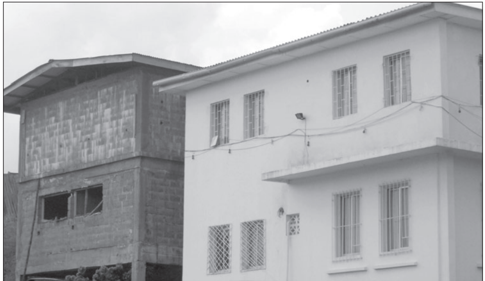
Figure 6: Liberian Ministry of Lands, Mines, and Energy Building and Secured Annex under Construction for Housing Liberia's Rough Diamond Exporting and Importing Authority
