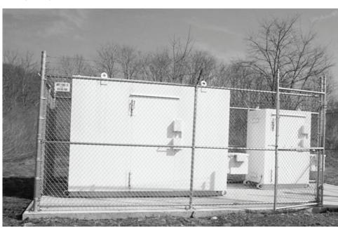
Figure 4: Pennsylvania Storage Facility with Interior Barrier Surrounding Type 2 Storage Magazines
