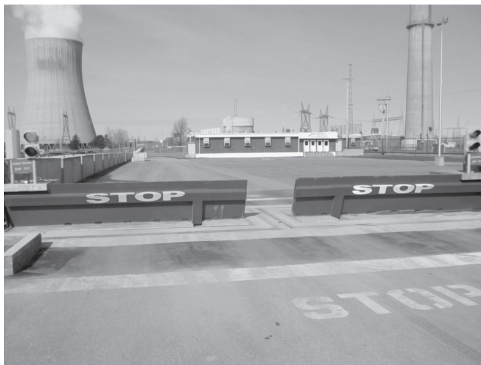
Figure 4: Example of an Active Vehicle Barrier System
