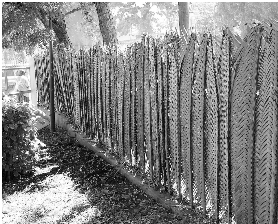
Figure 6: School Fence to Be Replaced under the Soft Targets Program
