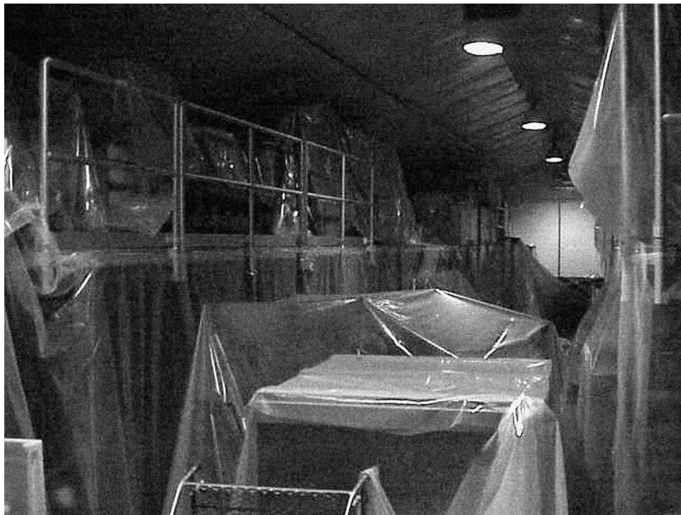
Figure 5: Measures to Shield Collections from Asbestos, Garber Facility, Suitland, MD
