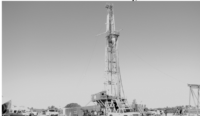
Gas Well Construction Site in Wise County, Texas
