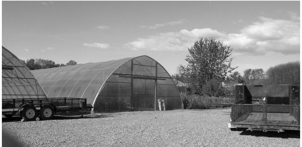
Figure 7: Example of Horticulture Enterprise EDA Funded
