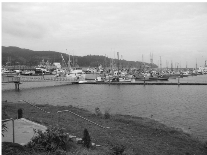
Figure 13: Marina and Breakwater Constructed with EDA Grant Funds
