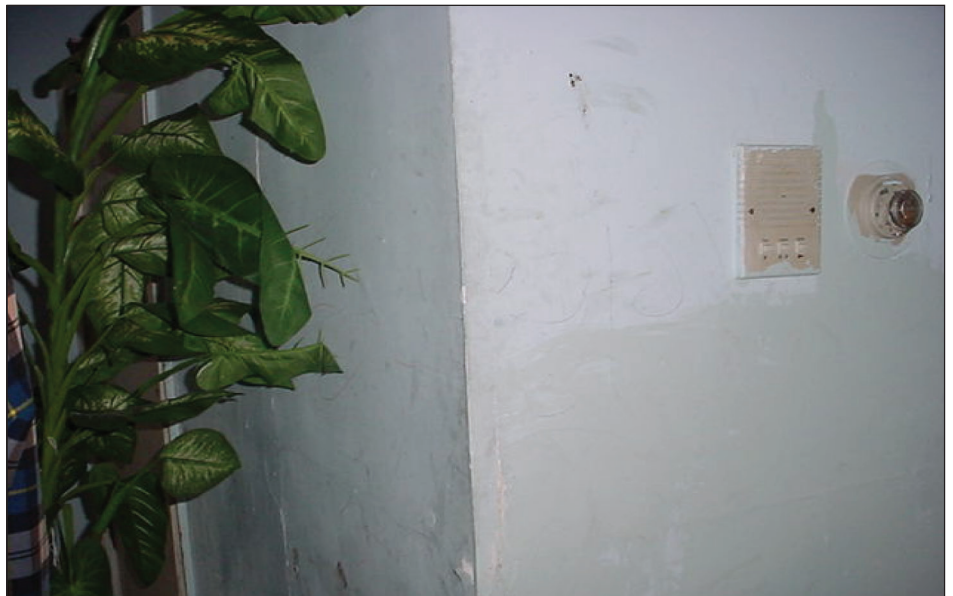
Figure 13: Property 1–“New” Sheetrock® Walls
