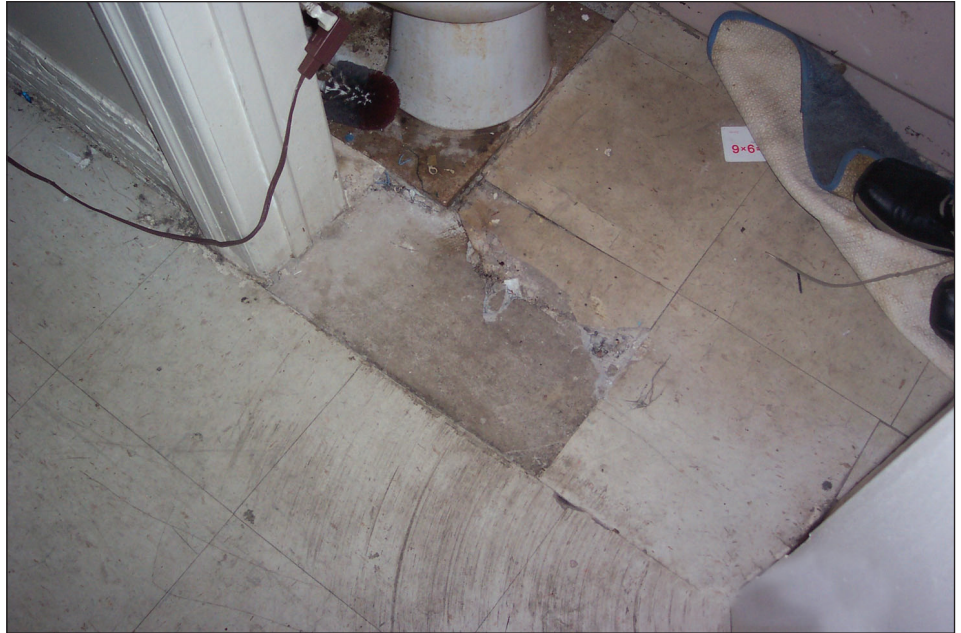
Figure 29: “New” Bathroom Floor
