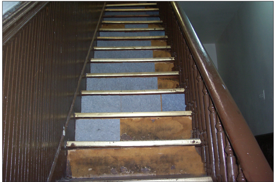
Figure 27: “Newly Tiled” Stairway
