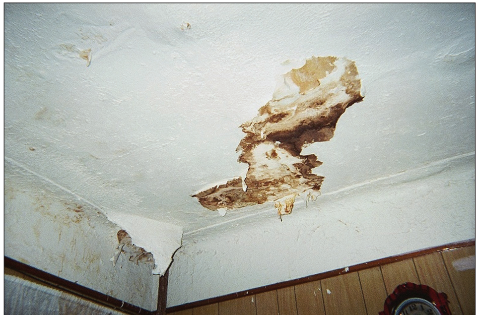
Figure 24: Property 5—"Plastered and Painted" Ceiling
