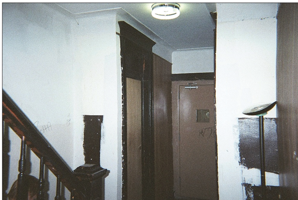
Figure 23: Property 5—“Repaired and Painted” Public Hall
