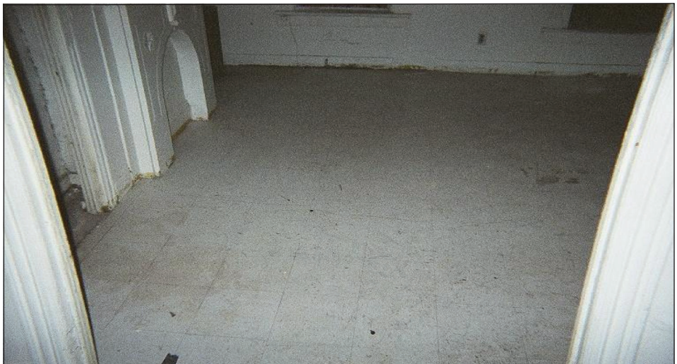
Figure 20: Property 3—"New" Living Room Floor
