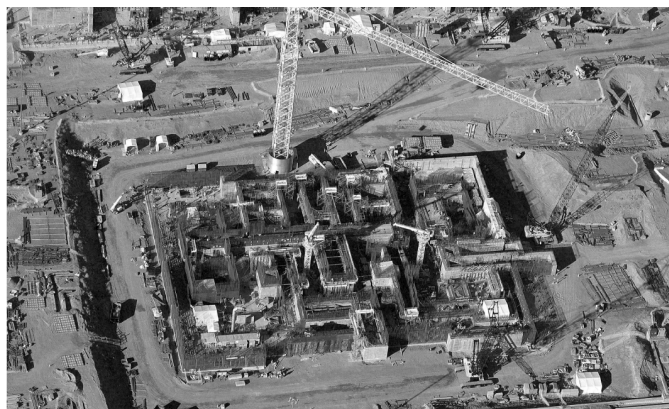
High-level Vitrification Plant at Hanford's Waste Treatment Construction Site, March 2004
