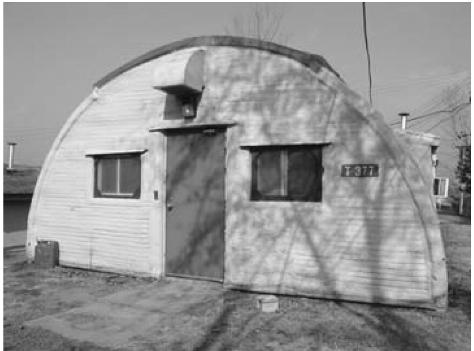
Figure 1: Quonset Hut Used for Barracks at Camp Greaves
