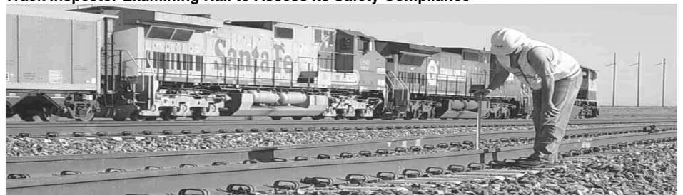
Track Inspector Examining Rail to Assess Its Safety Compliance
