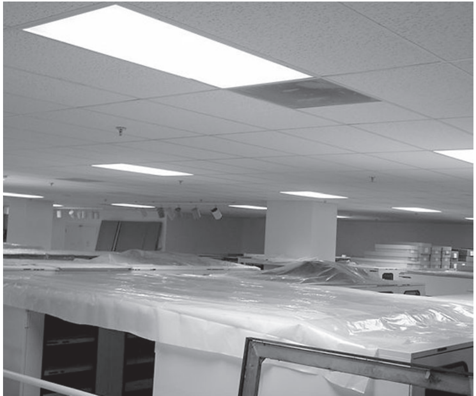
Figure 7: Plastic Sheetting Protecting Collection Items from Water Damage in a Storage Area of the Smithsonian Institution's Quadrangle Complex
