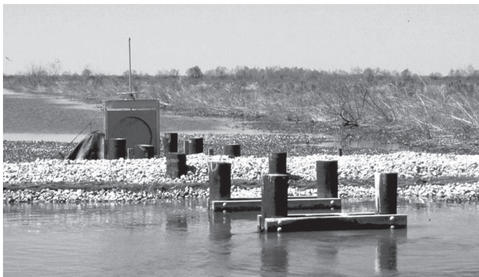
Figure 4: Gate in an Outfall Management Project
