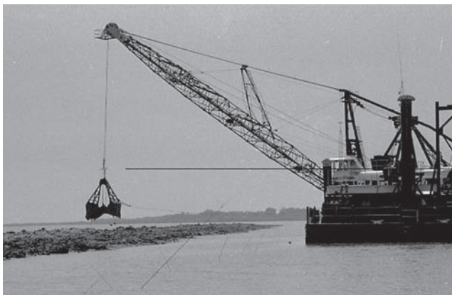
Figure 12: Constructing Terraces to Trap Sediment in Open Water
