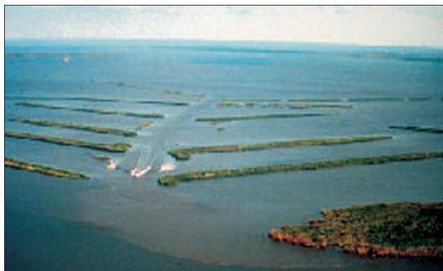
Figure 11: Terraces Built to Trap Sediment and Slow Water Flow
