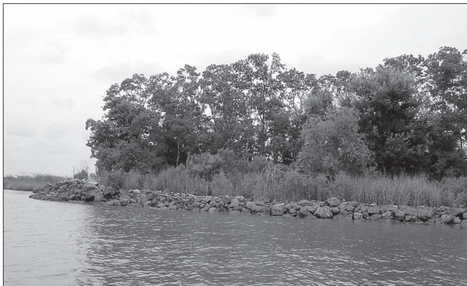
Figure 6: Rock Berm Built for Shoreline Protection
