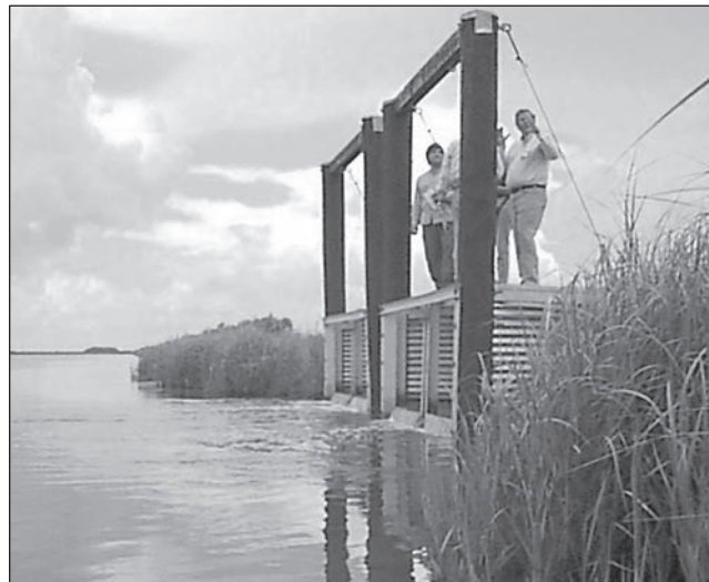
Figure 8: Gates to Control Saltwater Levels
