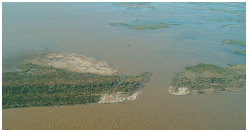
Figure 3: Crevasse in a Sediment Diversion Project
