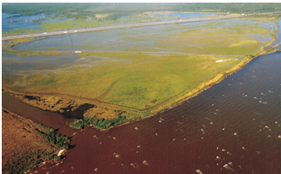
Figure 5: Marsh Creation Project Using Dredged Material
