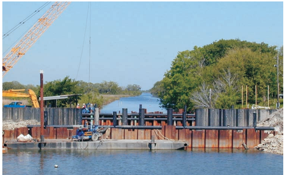
Figure 7: Water Control Structure to Restore Drainage Patterns and Water Flow
