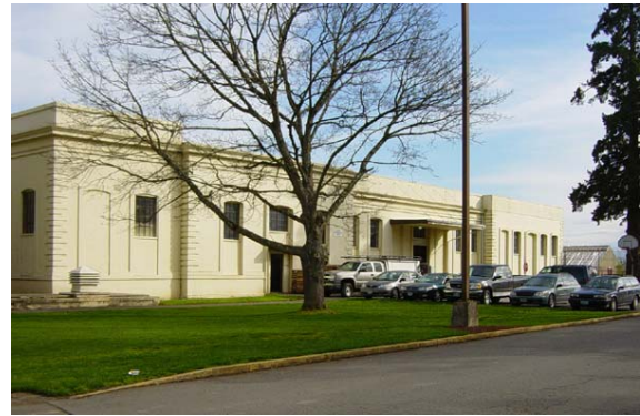
CENTRAL STORAGE, BUILDING 59
