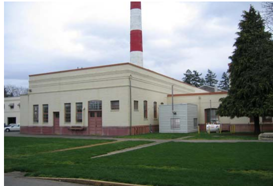
BOILER BUILDING, BUILDING 51
