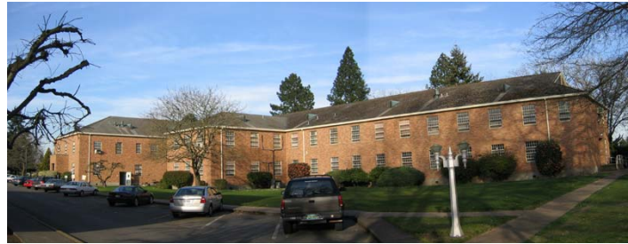
SANTIAM HALL, BUILDING 34
