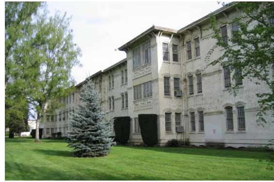
'J' COMPLEX, BUILDINGS 47/48
