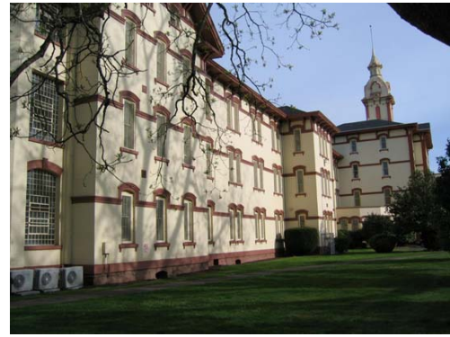
'J' COMPLEX, BUILDING 41
