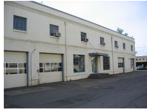
VEHICLE GARAGE, BUILDING 53
