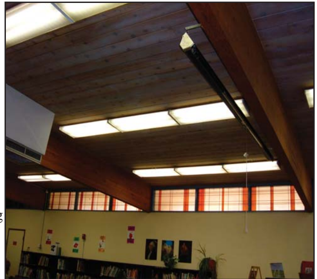
BEFORE - The library at Sunset Elementary School in Hermiston before the lighting update project is dark and had 73 fixtures. The district installed 80 new energy-efficient fixtures in the library and expects to save energy.
