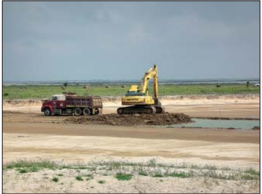
Heavy equipment operators remove excess material to create one of the channels connecting the three basins within the Babia Grande wetland complex, Texas. (Thor Lassen, Ocean Trust)
