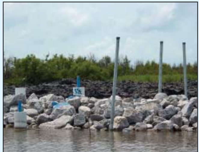
Typical view of geotechnical instruments (USACE).
