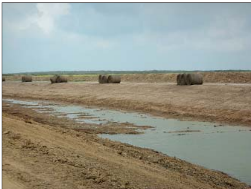
Native Gulf cordgrass lines the banks of the new channels and will be used to stabilize and enrich the soil, within the Babia Grande wetland complex, Texas. (Thor Lassen, Ocean Trust)
