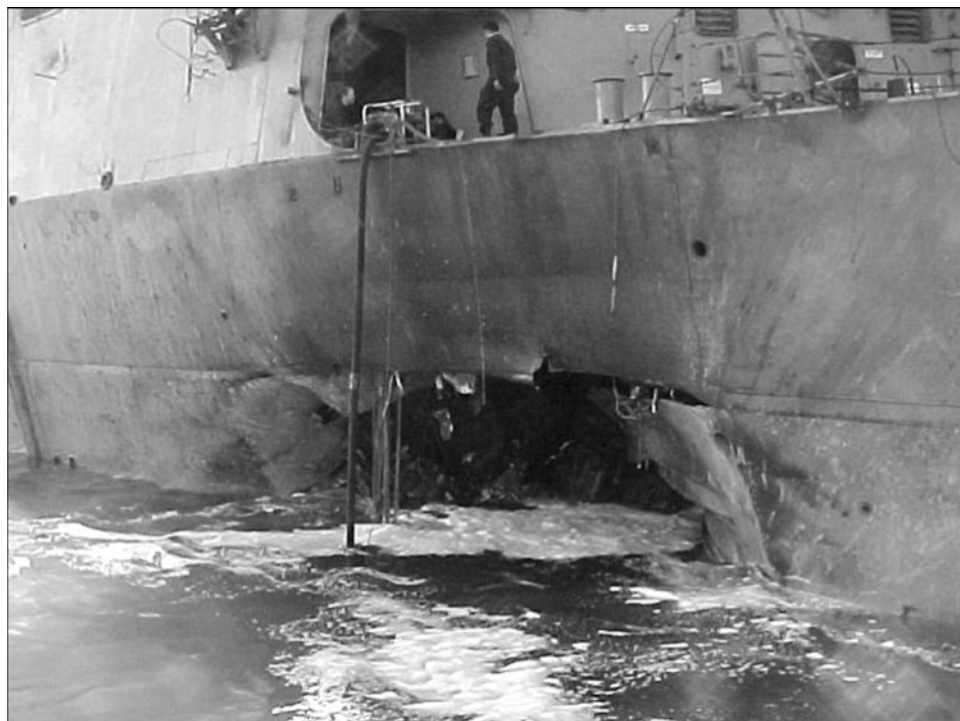
Figure 17: USS Cole Damaged by a Terrorist Bomb Explosion While Refueling at the Port of Aden, Yemen
