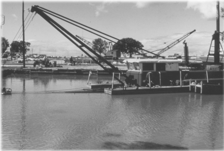
A contaminated sediment staging area.
