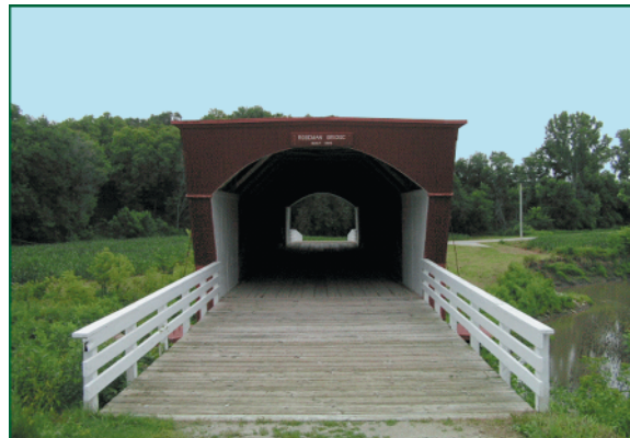
Roseman Bridge, Madison County, Iowa.
