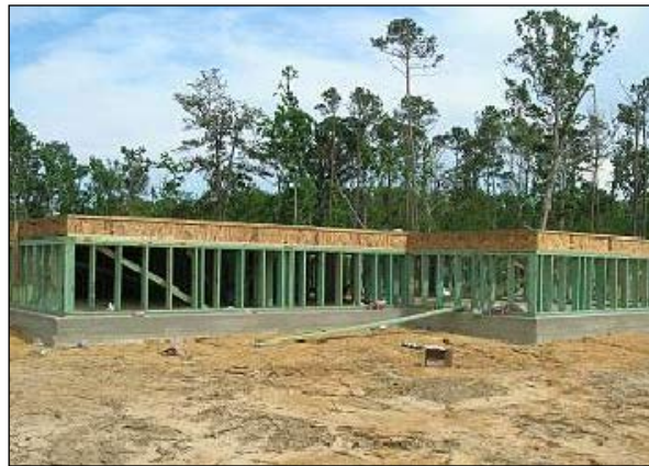
Raised wood floor on foundation walls.
