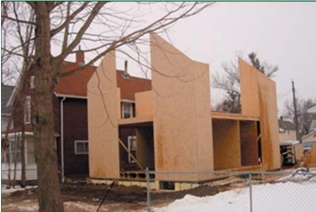
Using vertical SEP panels in construction of research house.
