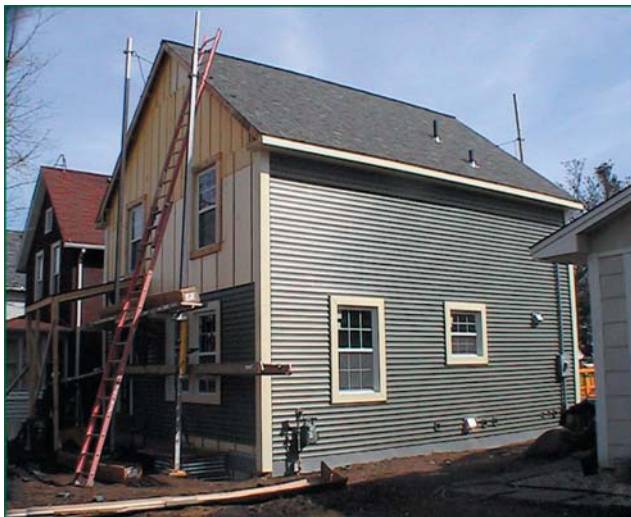
Completing the ETMMS and exterior finishes.
