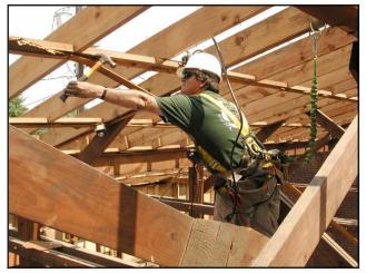
Dismantling buildings slated for demolition can provide a source of quality building materials. FPL researchers are testing the mechanical properties of reclaimed lumber and working to develop a grade stamp for the material.
