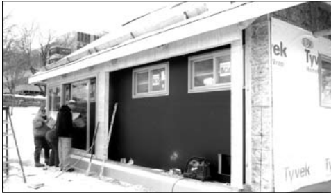
This interior wall, painted black and placed just inches behind two large windows, creates a “solar hot air collector,” maximizing the passive solar heating capacity of the Carriage House.
