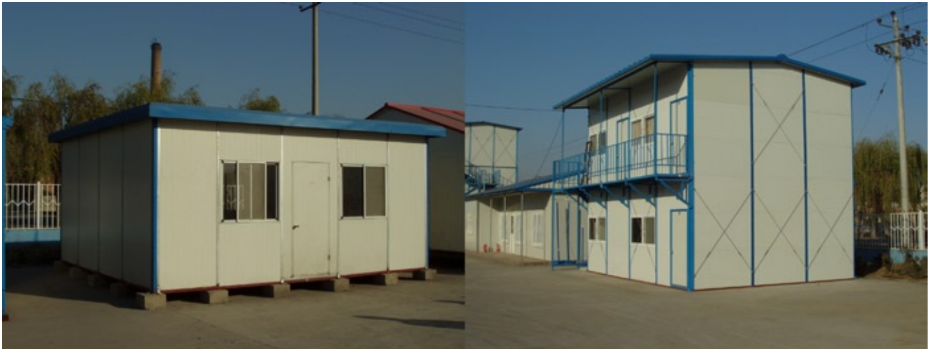
Figure 14—One- and two-story commercial steel buildings designed as site-assembled kits and made in China for use as temporary commercial and emergency structures.
