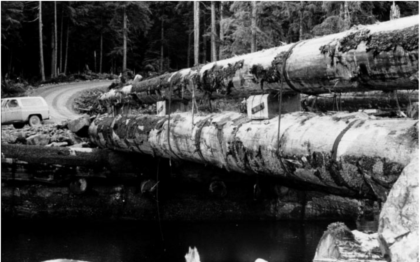
Figure 18–2. Logs are used to construct logging bridges in remote forest areas.
