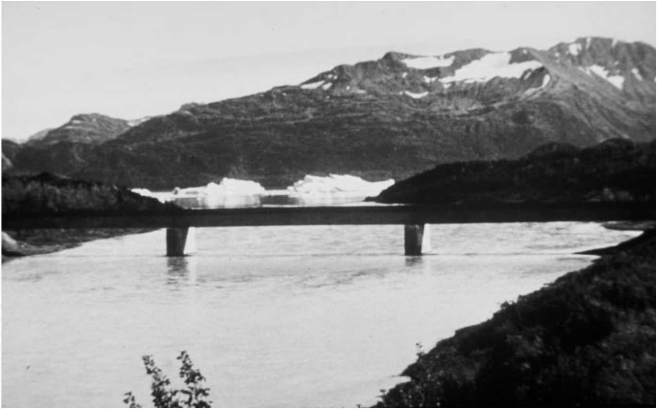
Figure 16–9. Glulam beam bridge over the Dangerous River, near Yukatat, Alaska, consists of three 43.5-m (143-ft) spans. Each span is supported by four 2.3-m- (91.5-in.-) deep glulam beams.
