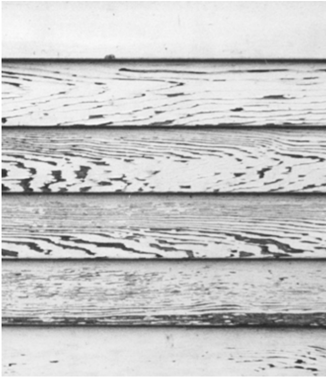
Figure 15-2. Paint applied over edge-grain boards (top and bottom) performs better than that applied to flat-grain boards (middle).
