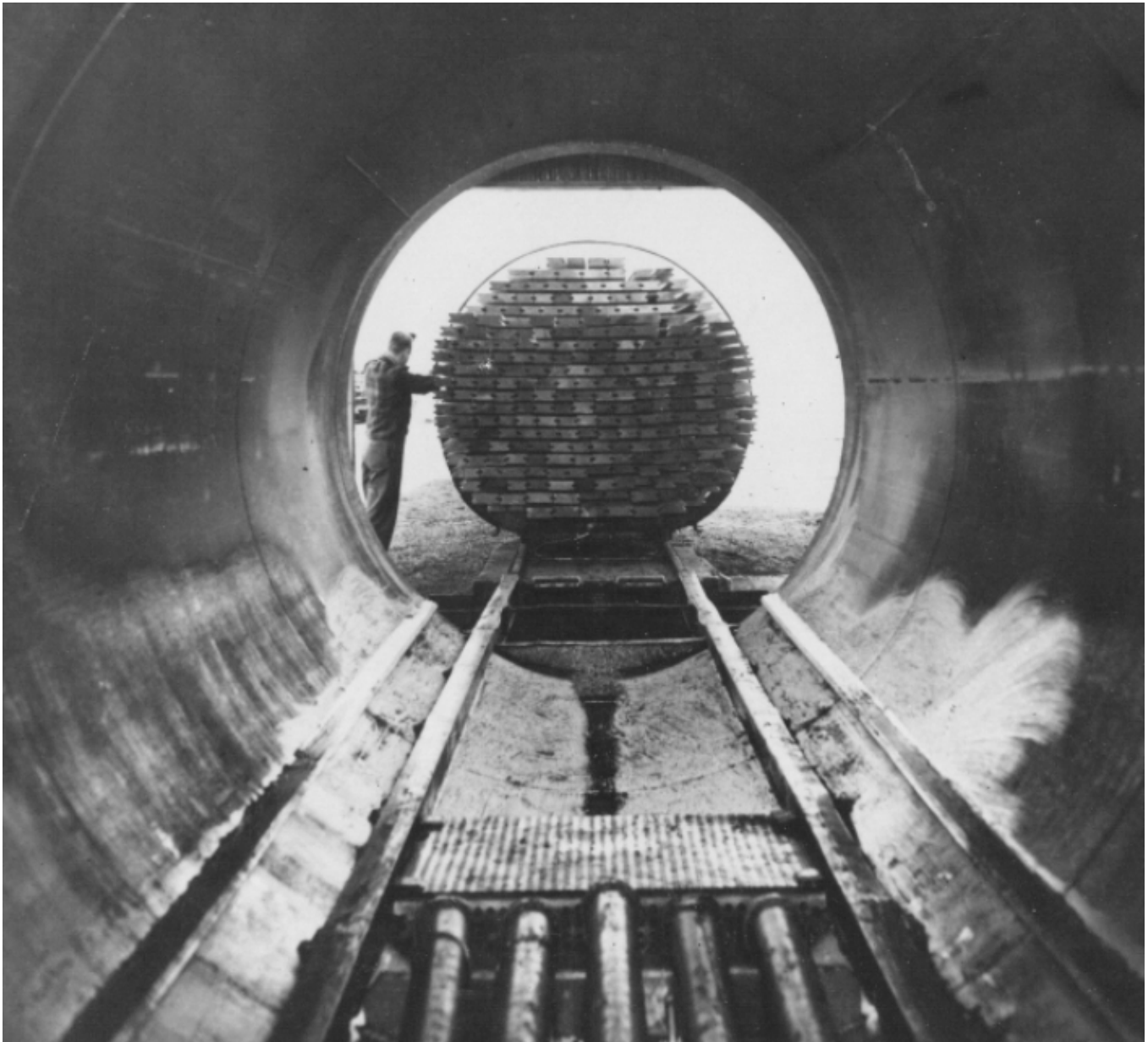
Figure 14-3. Interior view of treating cylinder at wood-preserving plant, with a load about to come in.
