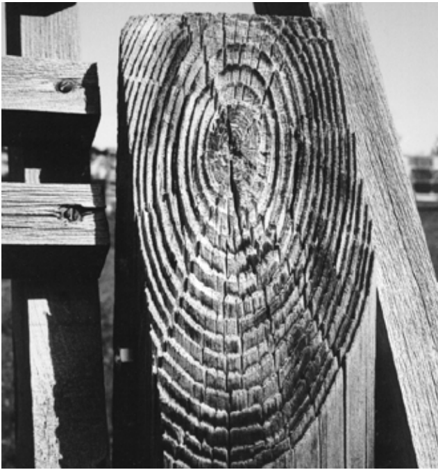
Figure 15–7. Weathered surfaces of softwood after 15 years of exposure in Madison, Wisconsin.
