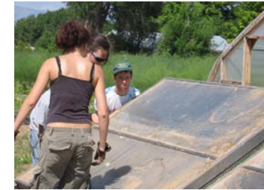
Workers help install solar panels.
