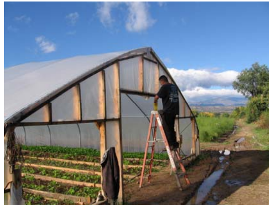
Greenhouses under construction at Santa Cruz Farm and Greenhouses
