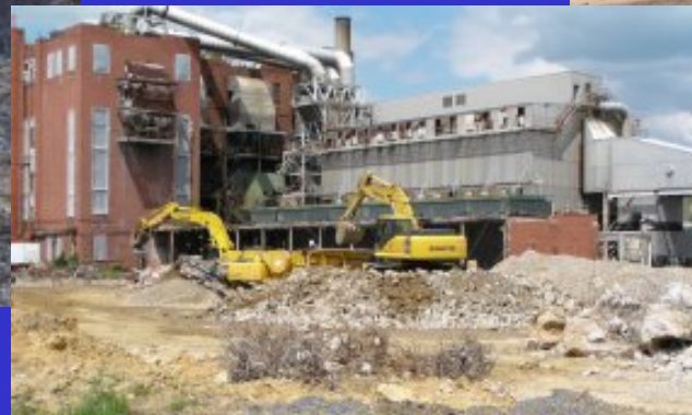
Avtex Plant demolition
