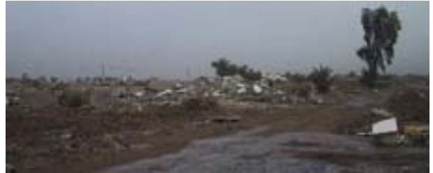
Destroyed Al Raya State Company.
