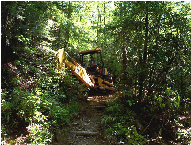
Figure 6. Backhoe working trail
