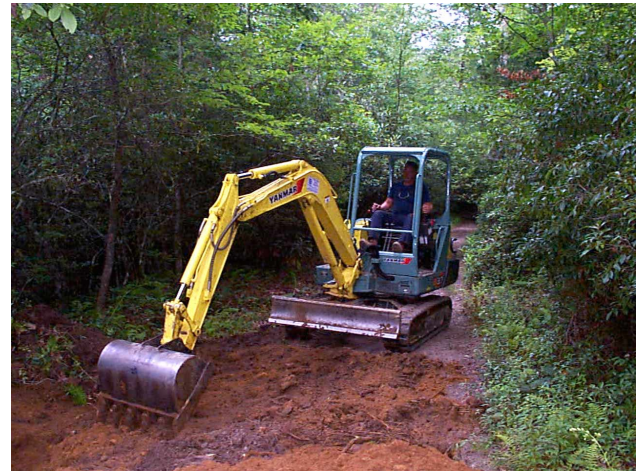
Figure 7. Mini-excavator working trail
