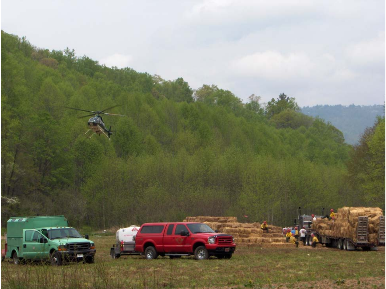
Helicopter Used to Seed, Fertilize and Mulch Landslides on the Grandfather District of the Pisgah National Forest
