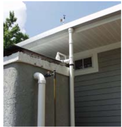
Cistern collects rain for nonpotable uses.
