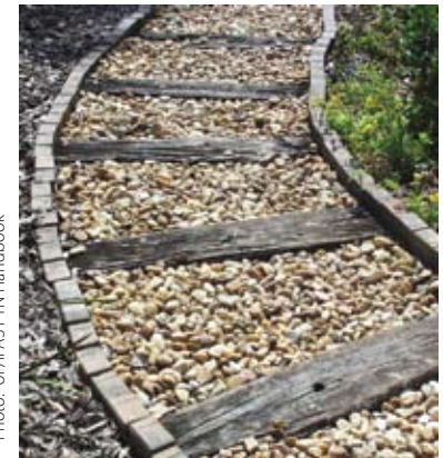
Recycled railroad ties, bricks and gravel make a unique footpath capable of absorbing rainwater.
