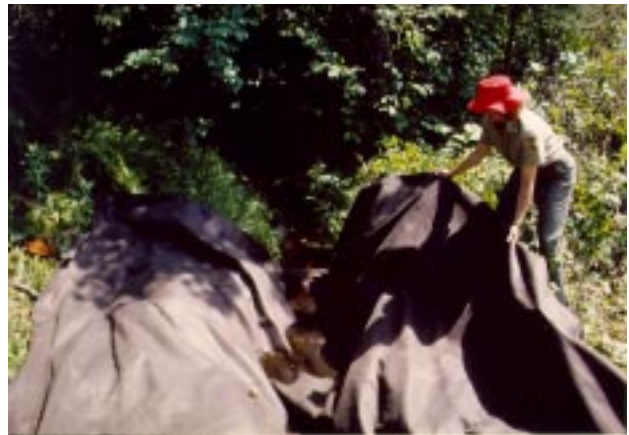
Figure 20.—Installation of a geotextile under a pipe bundle.
