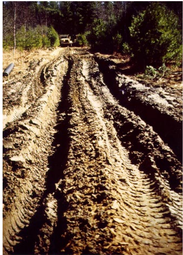
Figure 3.—Rutting that can occur when crossing soft, wet soils.
