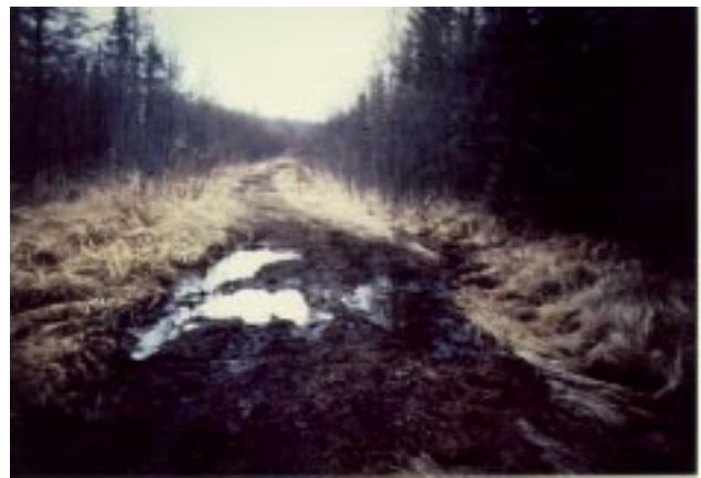
Figure 31.— Wet area in a haul road.
