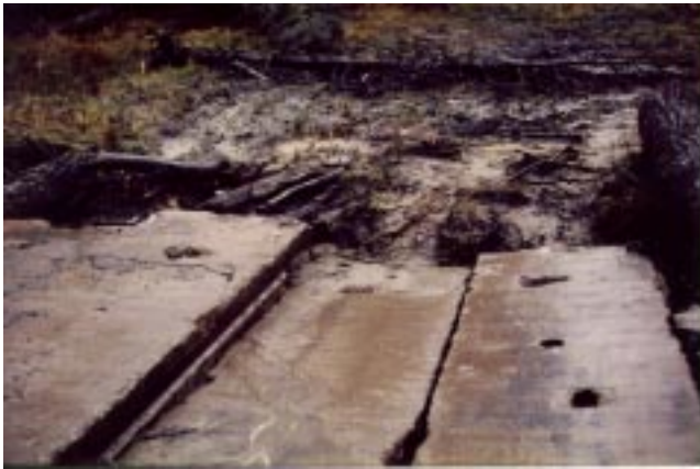
Figure 30.— Pre-stressed concrete bridge.
