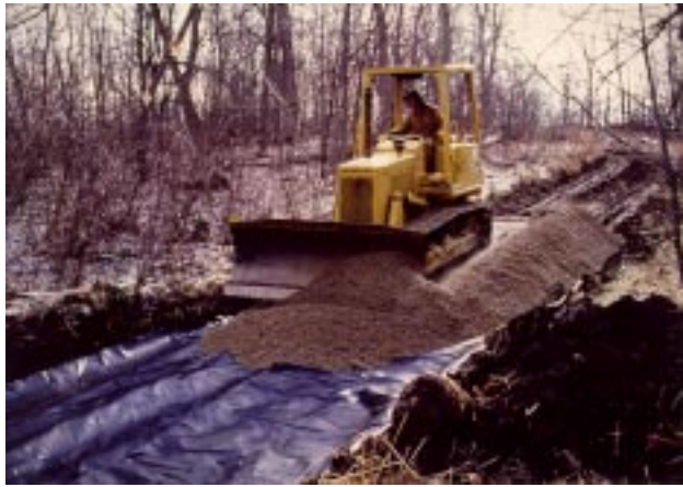
Figure 15.—A geotextile used in a ford.
