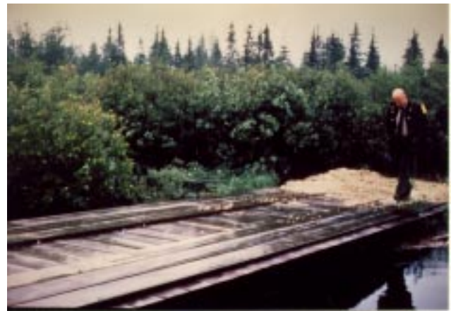
Figure 28.—Bridge made from a used railroad car.
