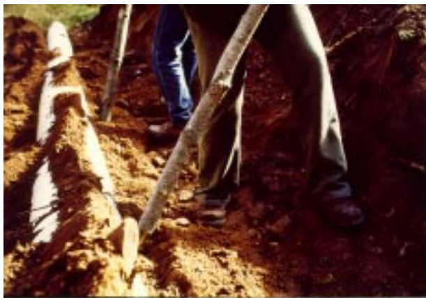
Figure 18.— Packing earth around a culvert during installation.
