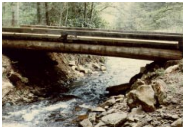
Figure 24.—Log stringer bridge.
