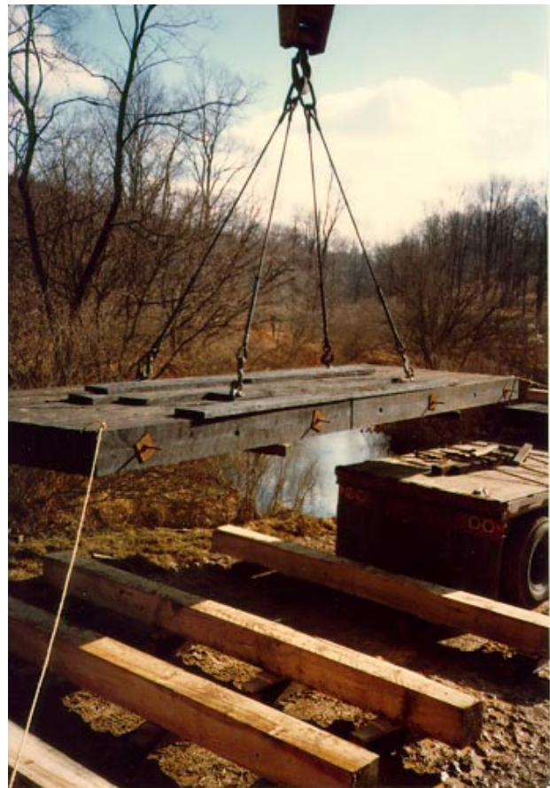
Figure 27.—Stress-laminated timber bridge panel.
