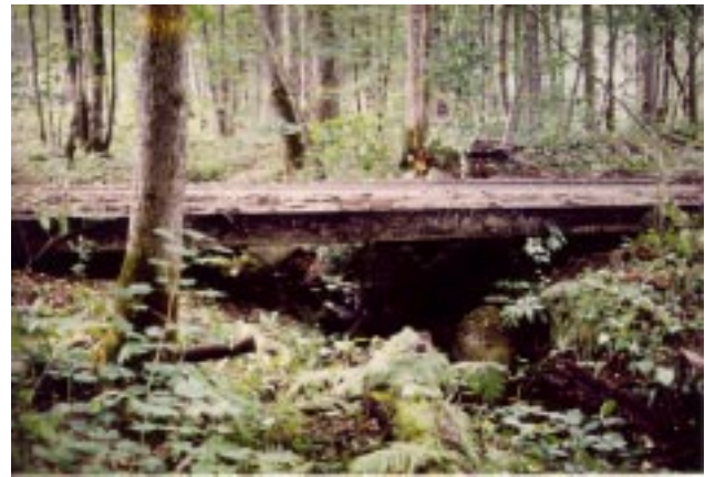
Figure 22.— Temporary bridge spanning a stream.
