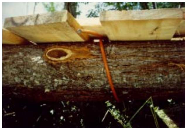
Figure 25.—Cabled logs in a log stringer bridge.
