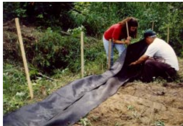
Figure 9.— Installation of silt fencing.
