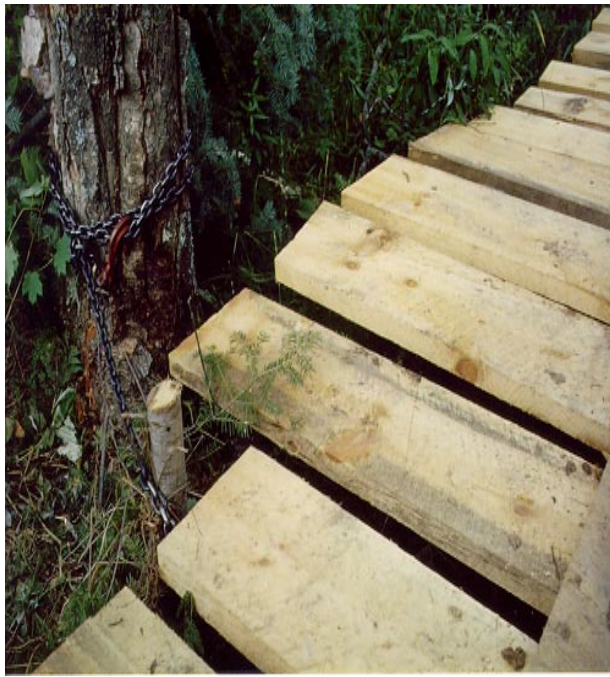
Figure 4.—Anchoring of a bridge to a nearby tree.
