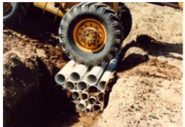
Figure 19.— PVC or HDPE pipe bundle.
