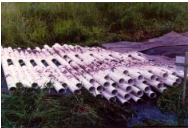
Figure 21.—Pipe bundle crossing layered to the desired height.
