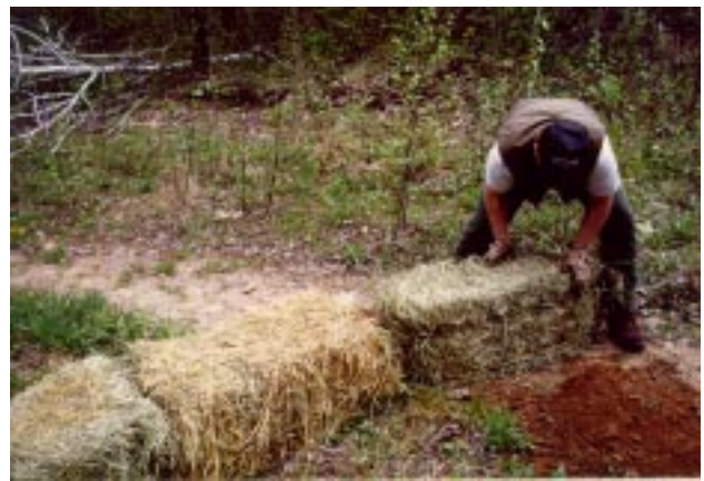
Figure 8.— Installation of hay or straw bale barriers.
