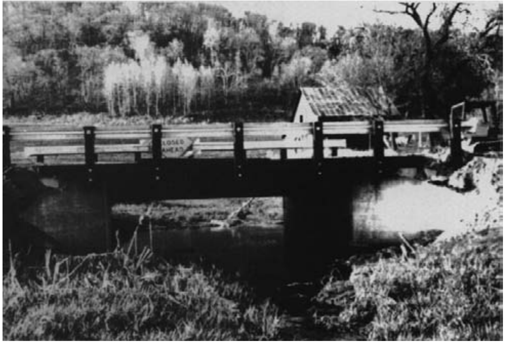
Figure 15-26. - The completed project with widened roadway, ready for paving.
