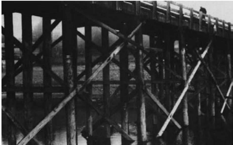
Figure 15-17. - Pile bents after replacement of deteriorated sections by pile posting.
