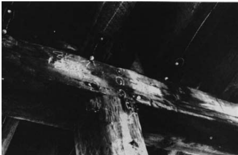
Figure 15-15 - Underside view of an intermediate bent cap after treatment was completed. Holes drilled for treatment application have been plugged with treated-wood dowels.
