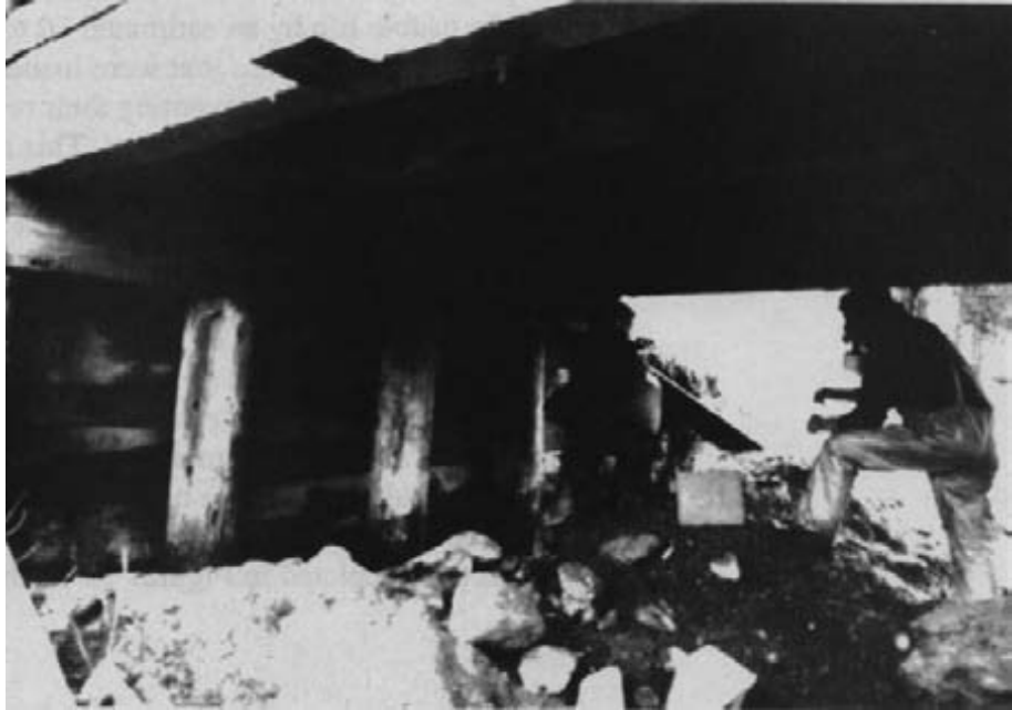
Figure 15-14. - Liquid fumigants being applied to the timber abutment.
