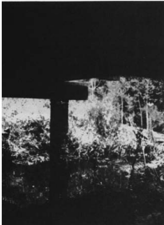
Figure 15-4. - Completed pile posting with protective plastic in place.
