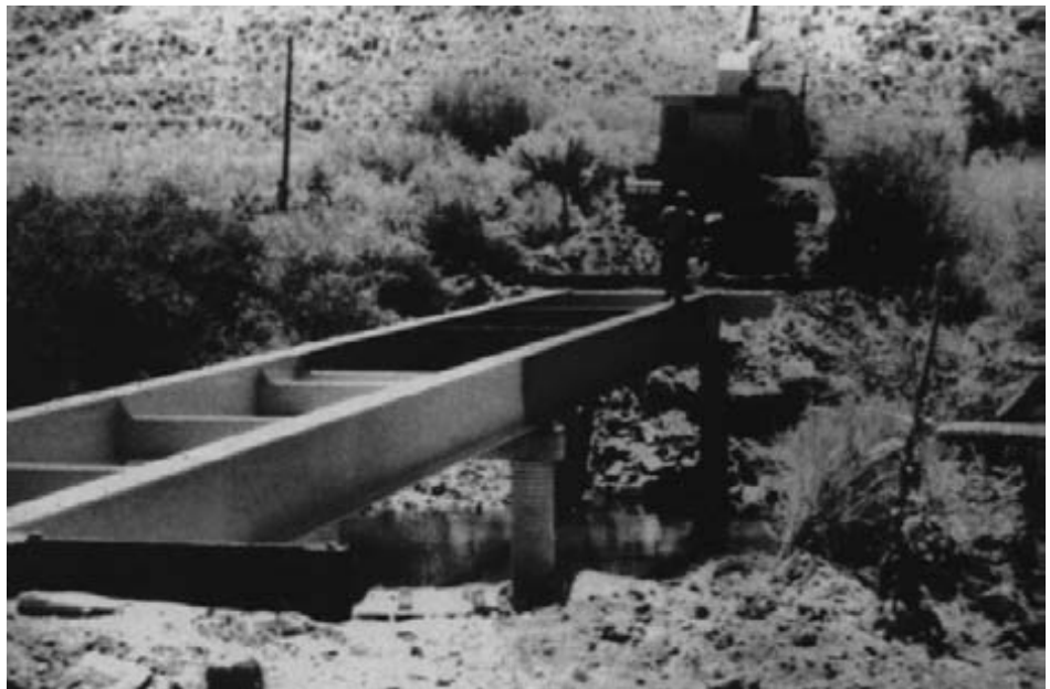
Figure 15-61. - Steel beam extensions in place and pinned to the existing beams.
