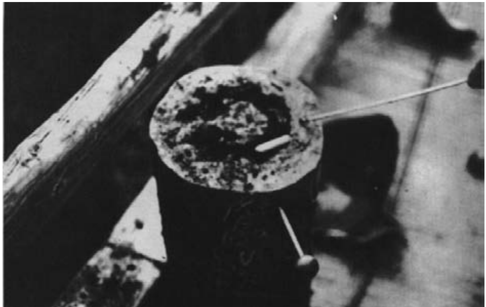
Figure 15-2. - Section of deteriorated pile removed from the structure.
