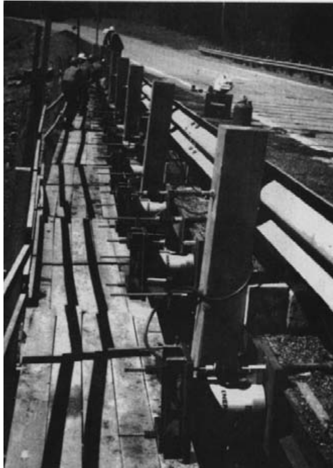
Figure 15-44. - Multijack hydraulic system used at the North Pagwachuan River Bridge.
