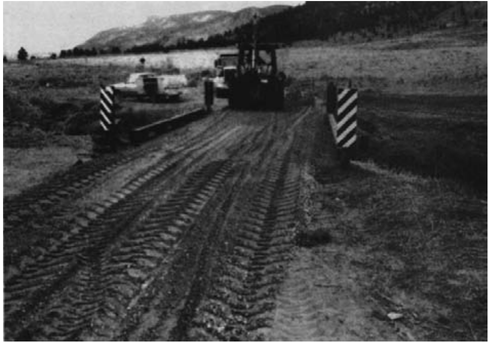
Figure 15-75. - The completed structure with a temporary aggregate wearing surface. The deck was later provided with an asphalt pavement wearing surface.
