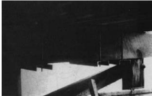
Figure 15-45. - Tie-down of the deck to supports at the Kabaigon River Bridge.
