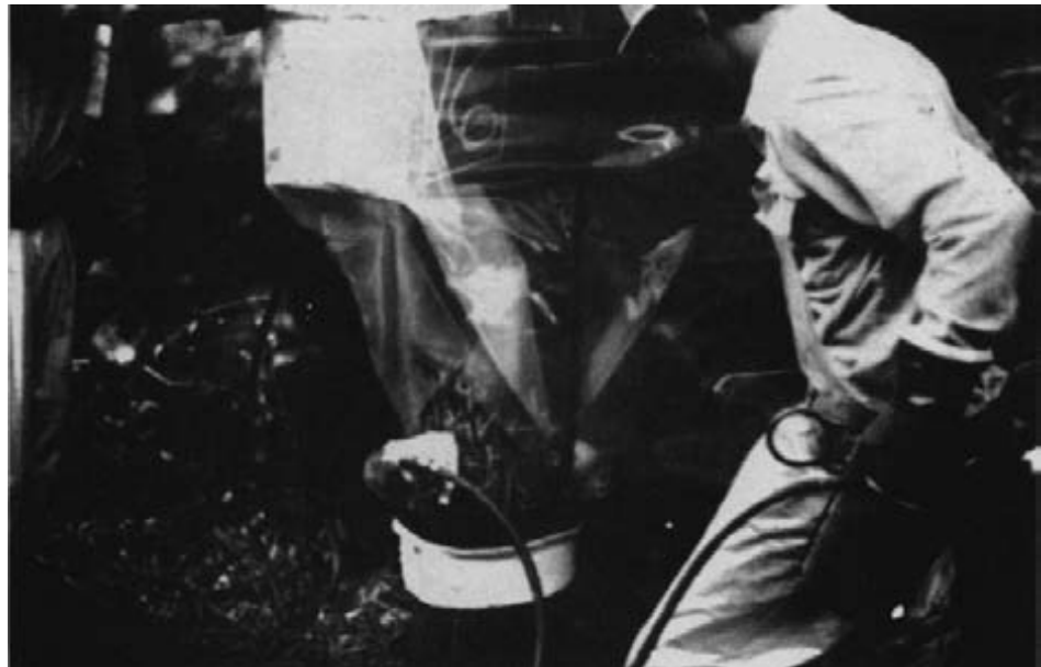
Figure 15-9. - Injection of liquid preservative solution into a timber pile.
