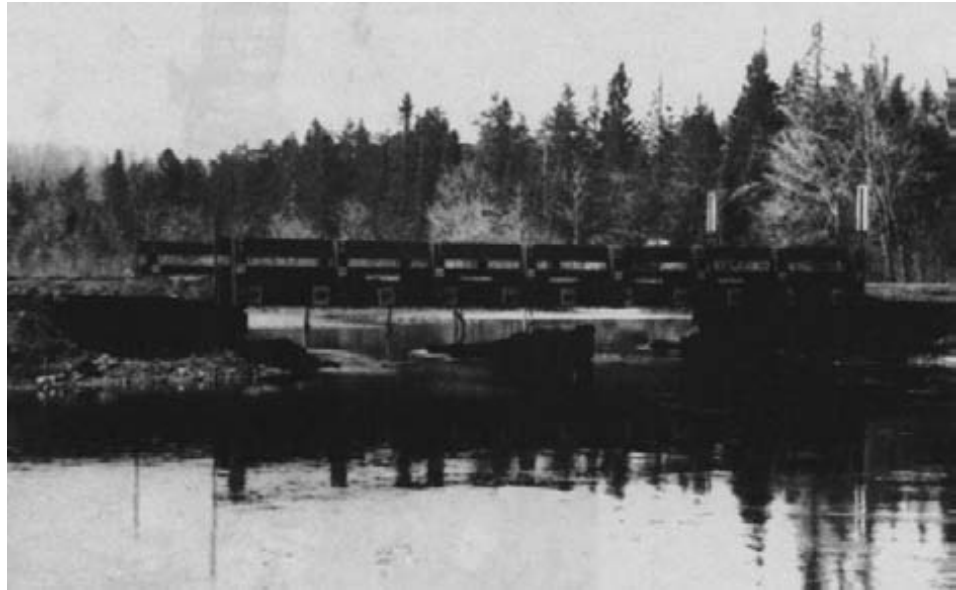
Figure 15-81. - The completed longitudinal stress-laminated deck bridge replaced the existing two-span structure with a single span. The new deck increased load capacity to AASHTO HS 20-44 and included curbs and railing. Remains of the old center support are visible below the replacement structure (photo courtesy of Wheeler Consolidated, Inc.).
