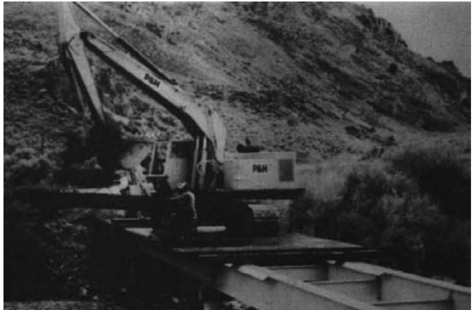
Figure 15-63. - Transverse glulam deck panels are lifted into place.
