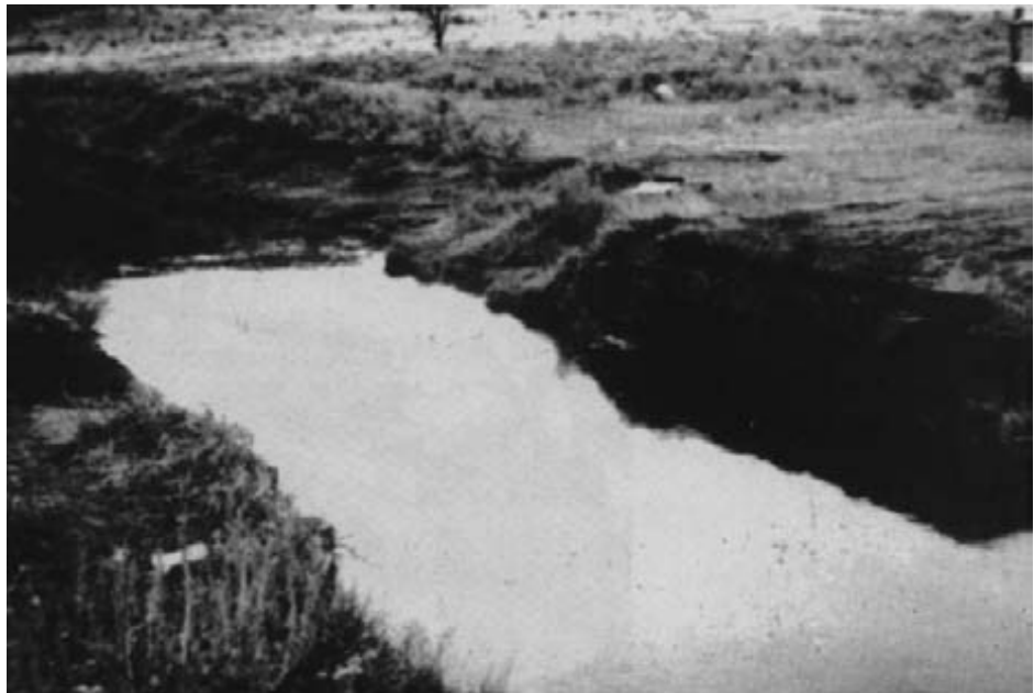
Figure 15-68. - A view of the abutments after the bridge was removed.
