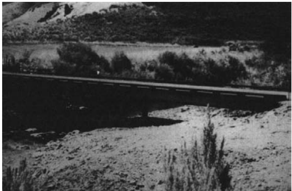
Figure 15-65. - The completed bridge with glulam curb/wheel guards and asphalt wearing surface in place.
