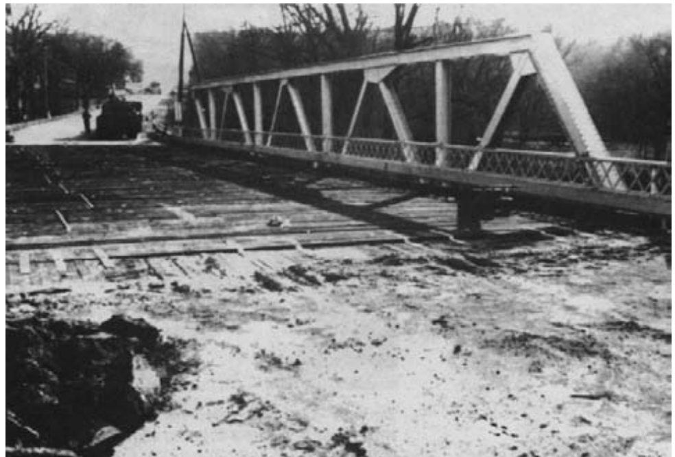
Figure 15-54. - The completed treated-timber deck, before placement of an asphalt-pavement wearing surface.
