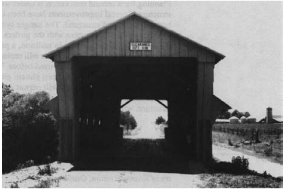
Figure 15-36. - The final result of the bridge-within-a-bridge concept. Four kneebraces to the roof system, which had been removed over the years, were reinstalled for stability and appearance. Note the improved truss alignment.
