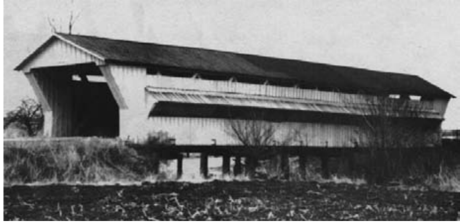
Figure 15-28. - Another view of the bridge before rehabilitation. One objective of the project was to maintain the bridge's appearance.
