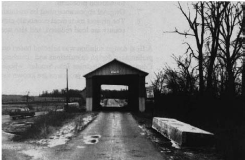
Figure 15-27. - Covered bridge on Winget Road before rehabilitation work began. Note the excessive rack and twist of the truss.
