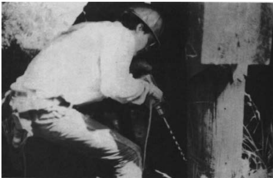
Figure 15-5. - Drilling holes for solid preservative cartridges.
