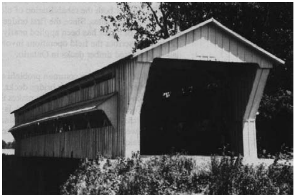
Figure 15-37. - The completed rehabilitation results in a significantly increased load capacity (18 tons), while maintaining the historic bridge's aesthetic appeal.
