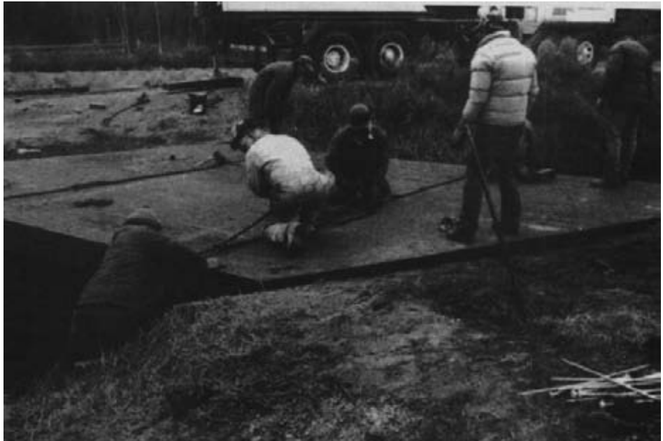
Figure 15-73. - The replacement deck in place.
