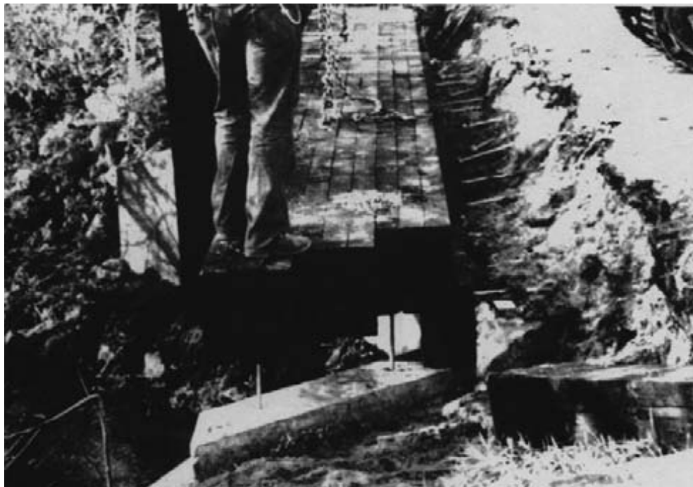
Figure 15-24. - A panel is lowered over the anchor bolts.
