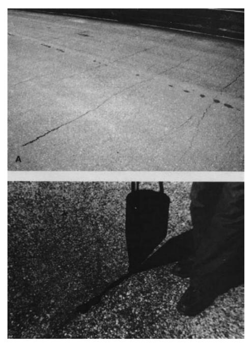
Figure 14-4. - (A) Minor cracking in an asphalt wearing surface from differential deck deflections. (B) Sealing the cracks with an asphalt emulsion slurry.
