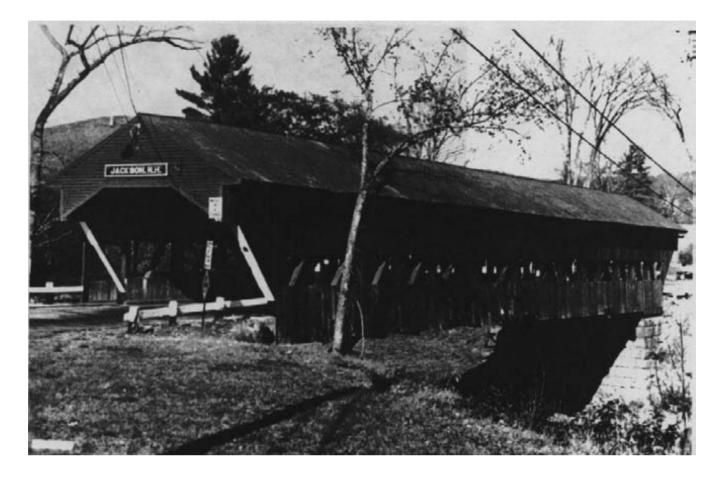
Figure 14-1. - Many covered bridges constructed of untreated timber, such as this one in New Hampshire, have lasted more than 100 years because they were protected from moisture.
