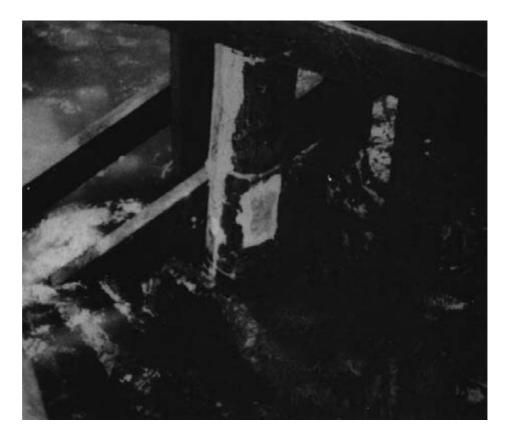
Figure 14-15. - Epoxy gel surface repair of a timber pile (photo courtesy of Osmose Wood Preserving, Inc.).
