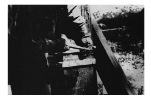
Figure 14-18. - A joint for a posting-type epoxy repair is sealed with plastic wrap stapled to the members. Small wood strips are then nailed across the plastic to provide an additional seal (photo courtesy of Osmose Wood Preserving Inc.).
