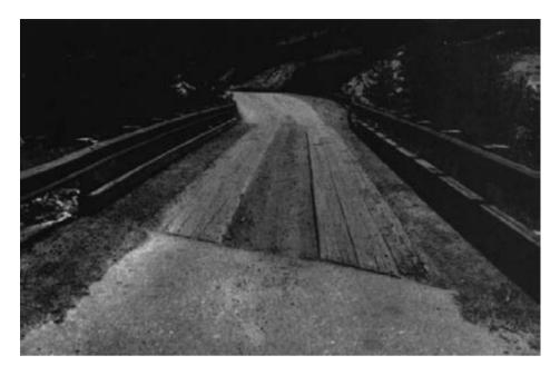
Figure 14-2. - Dirt and debris on the deck surface can trap moisture and lead to premature deterioration. Material such as this should be removed periodically as part of a good preventative maintenance program.
