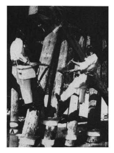
Figure 14-9. - Application of liquid fumigants. (A) Liquid fumigants applied with commercial equipment (photo courtesy of Osmose Wood Preserving, Inc.).
