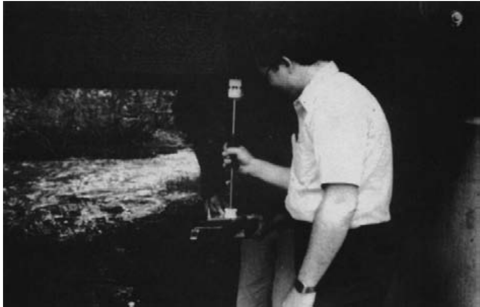
Figure 13-44. - The moisture content of a timber beam is measured with a resistance-type moisture meter.
