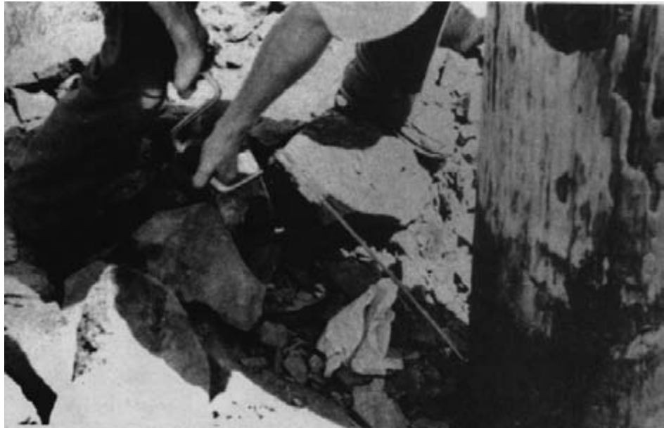
Figure 13-41. - Hand drilling at the base of a timber pile.
