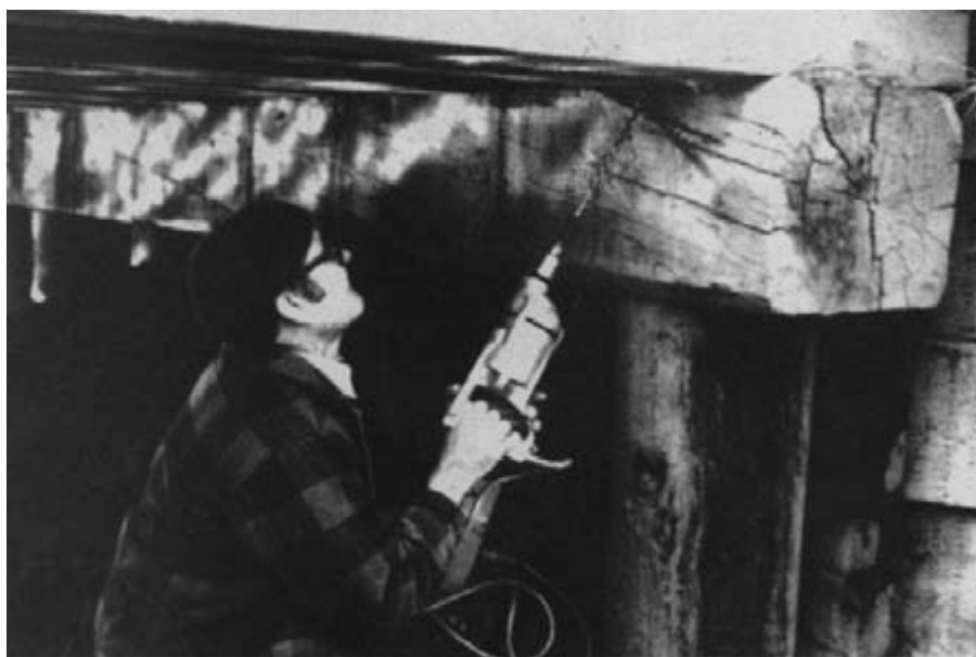
Figure 13-28. - Drilling the underside of a timber bridge beam to detect internal voids. The inspector feels and listens for torque release as the drill bit enters the wood, and examines shavings for evidence of decay.
