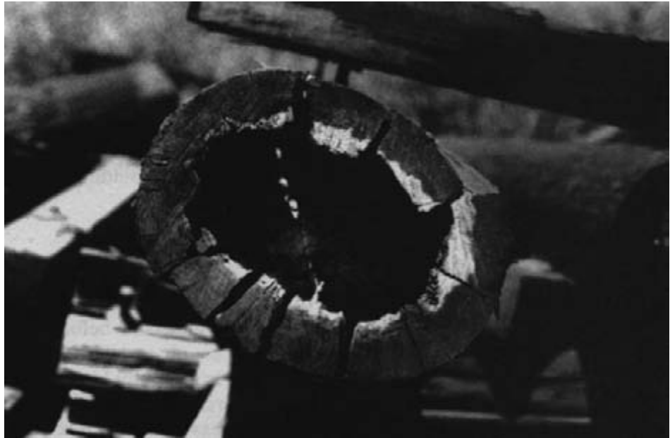
Figure 13-43. - Internal decay in a timber pile where it was drift-pinned to the cap. Before the breakage of the outside shell, caused by cap removal, the pile showed little exterior sign of the interior decay.
