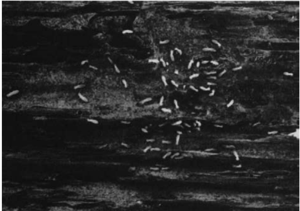
Figure 13-9. - Subterranean termites and the wood damage they cause. Note the frass and debris accumulations in the tunnels (photo courtesy of USDA Forest Service, Forest Sciences Laboratory, Gulfport, Mississippi).
