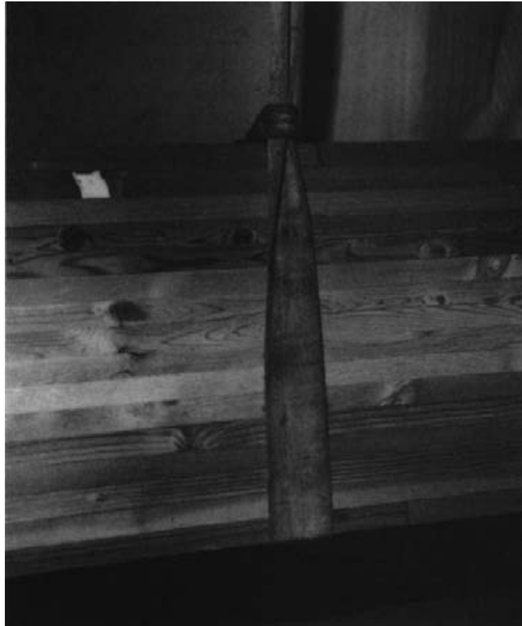
Figure 12-6. - Proper placement of a nylon sling on a glulam beam, with the loop in the sling at the corner of the beam.
