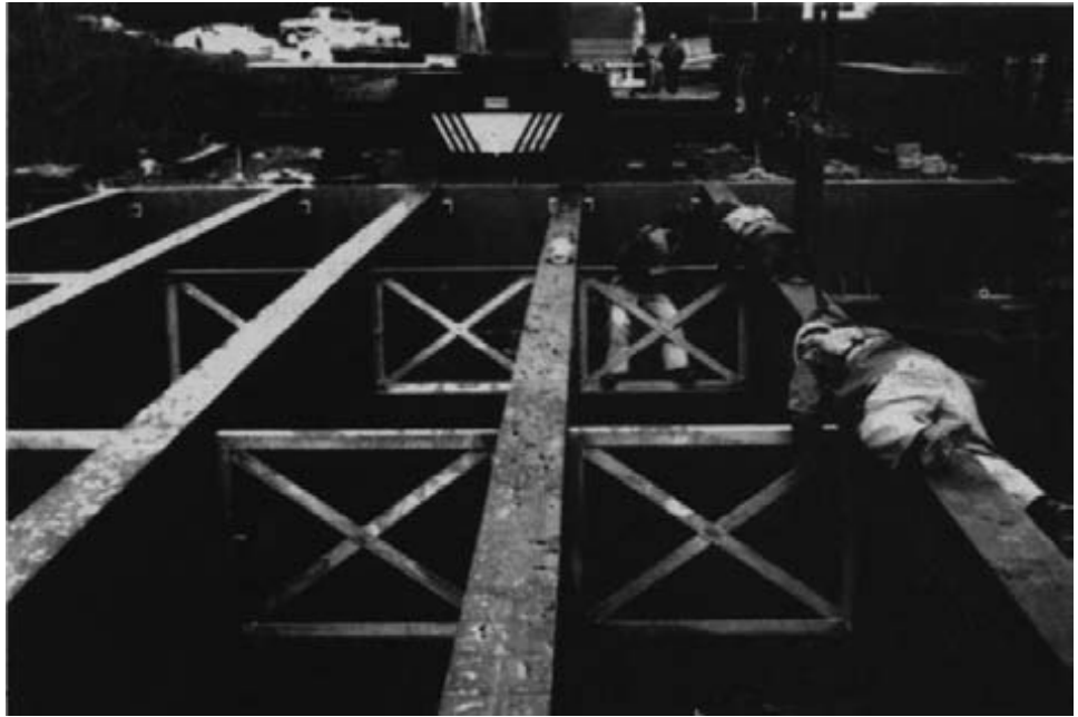
Figure 12-14. - Glulam beams for this bridge are placed from left to right, starting with the outside beam. As the beams are placed in position, bolts are inserted through bearings and steel cross-frames (photo courtesy of Western Wood Structures, Inc.).
